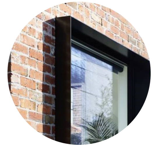
Metal Framing 'Monument' or similar colour as an added feature in the lower podium area around windows and archways.
