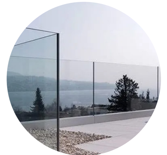
Glass Framless Balustrading Balustrading to Northern Podium to be framless to reduce its visual bulk and blend with the surrounding vegetation
