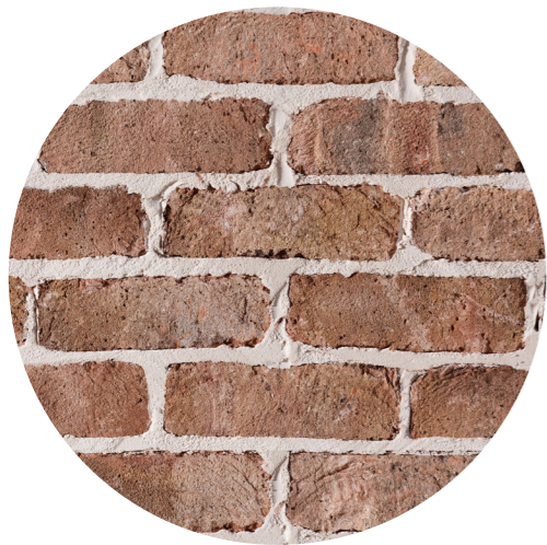
Face Brick Robertsons Rustic Face red bricks at ground floor podium along West and South laneways
