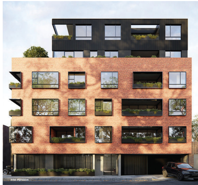
Brickwork – continuation of materiality from adjacent historic building in a contemporary form
