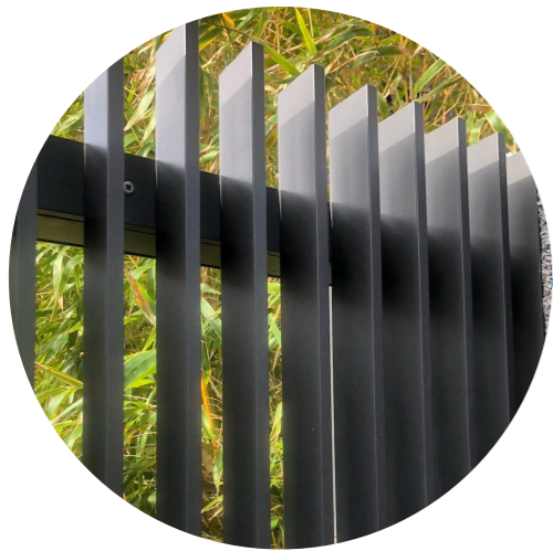
Vertical Monument metal balustrading to level 1 balconies designed to create architectural variety between podium and tower.
