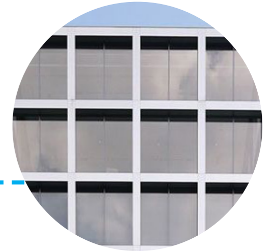
Grids in the podium façade reference the articulation from the adjoining historical building.
