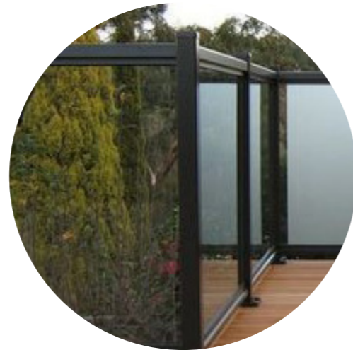
Glass Balustrading Balustrading to tower to be Monument aluminium framed with Glass infills creating continuity in tower finishes.
