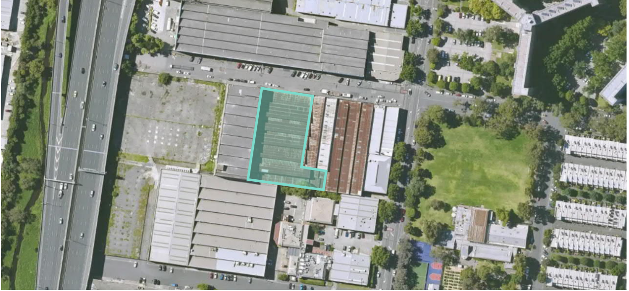
Figure 2: Aerial view of 77-83 Sutton Street, North Melbourne (Source: Landchecker, Markup by SDC)
