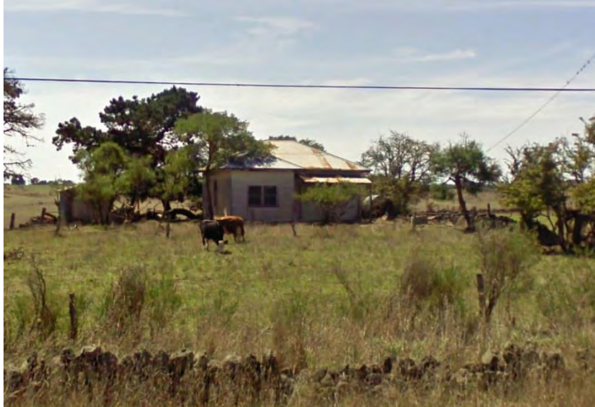
Figure 17 – Unoccupied and dilapidated house on Ondit-Warrion Road
