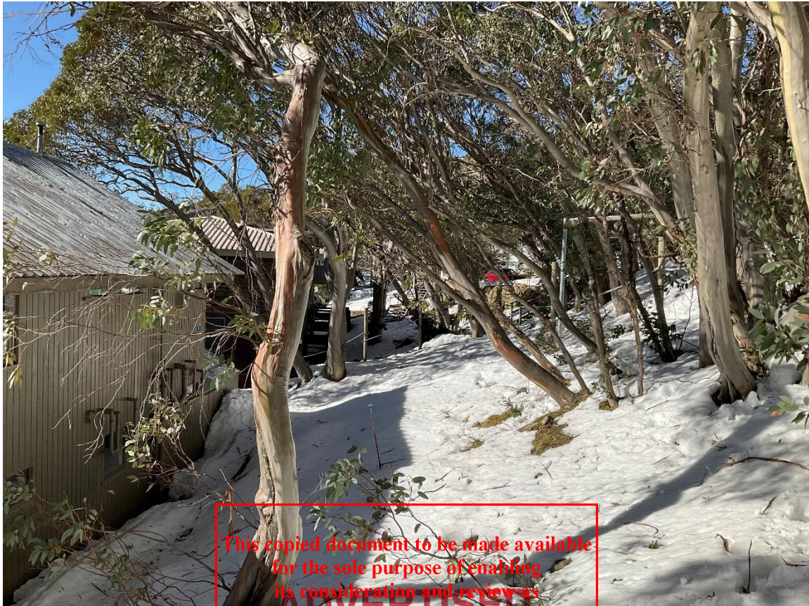
South of building
