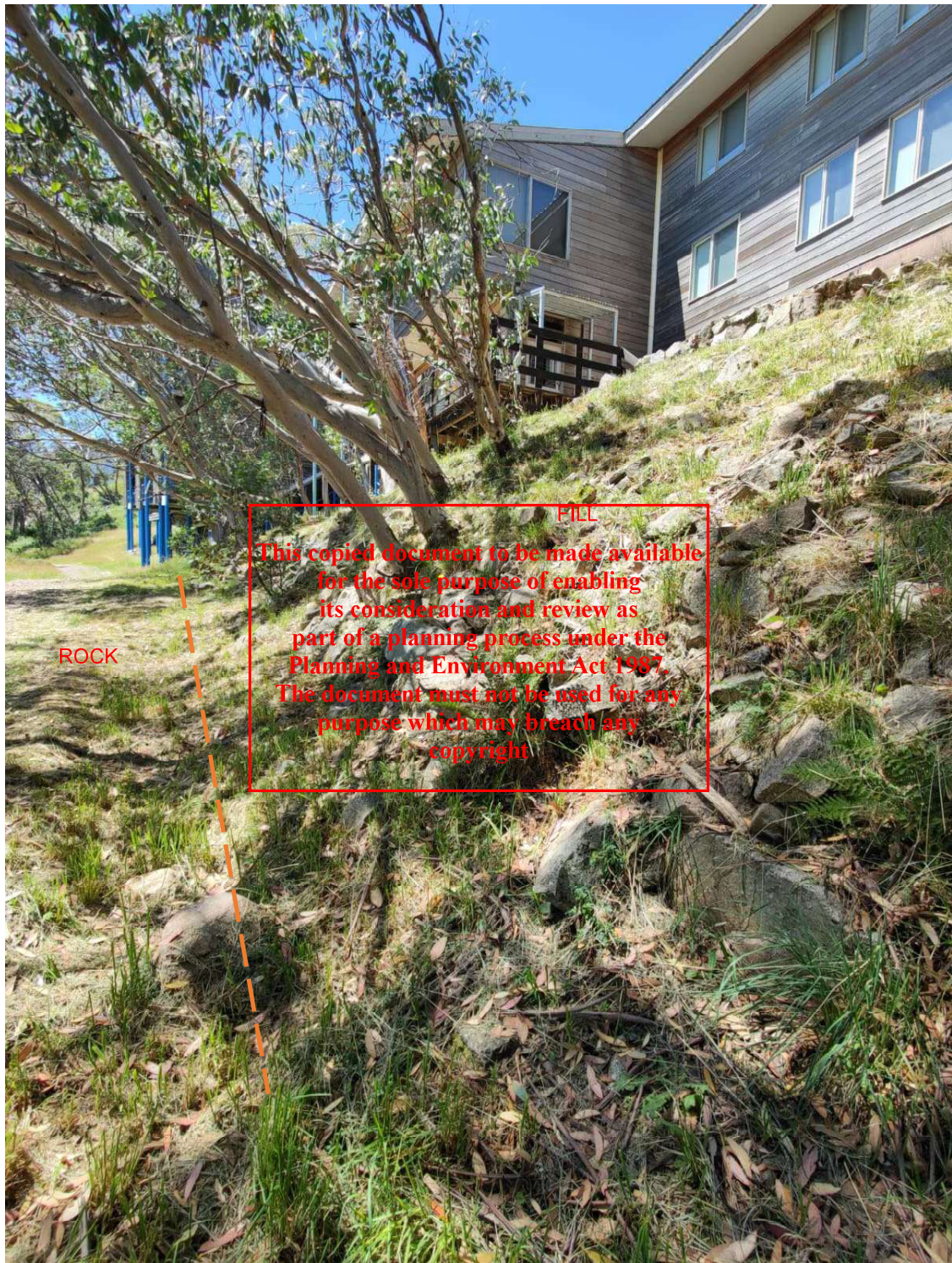
Plate 7. Northern side of property looking east with rock'/fill interface shown.
