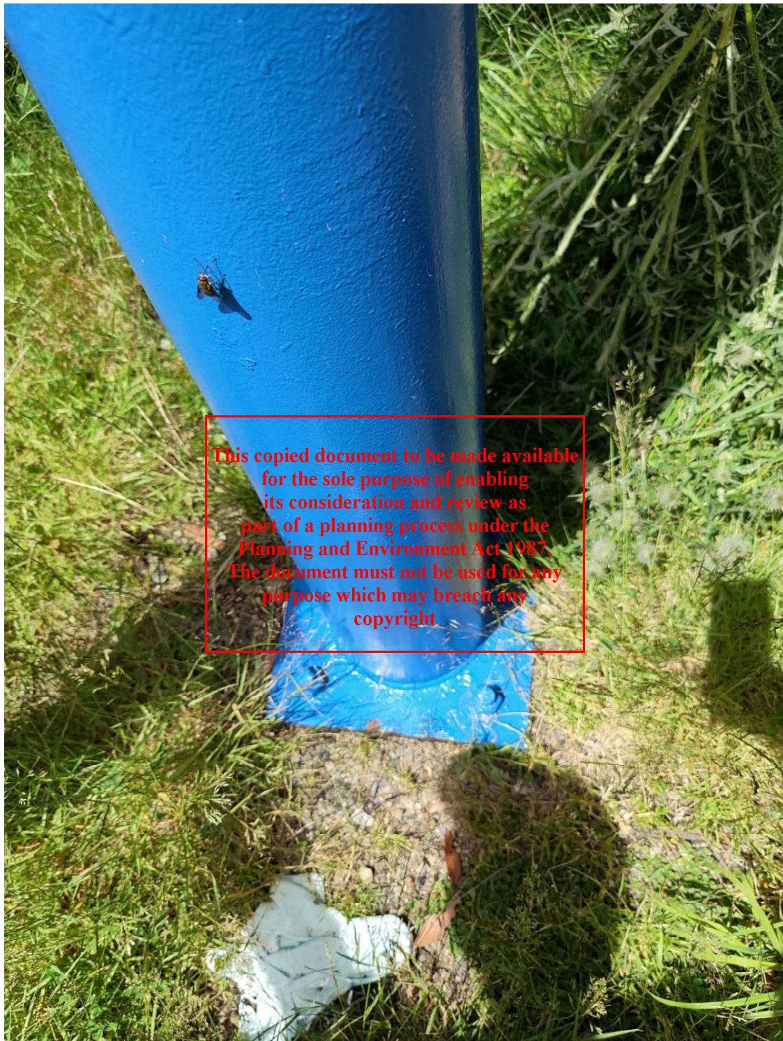
Plate 8. Balcony support on adjacent CSIR Lodge bolted into rock.
