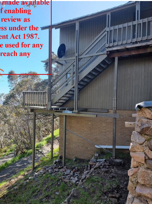
Non compliant escape stair-west elevation
