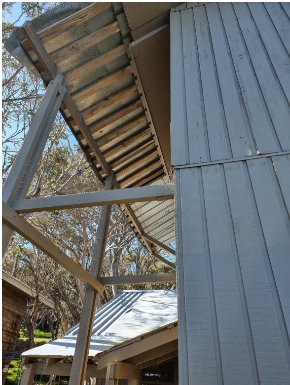
Typical non compliant roof and eaves/verandah overhang
