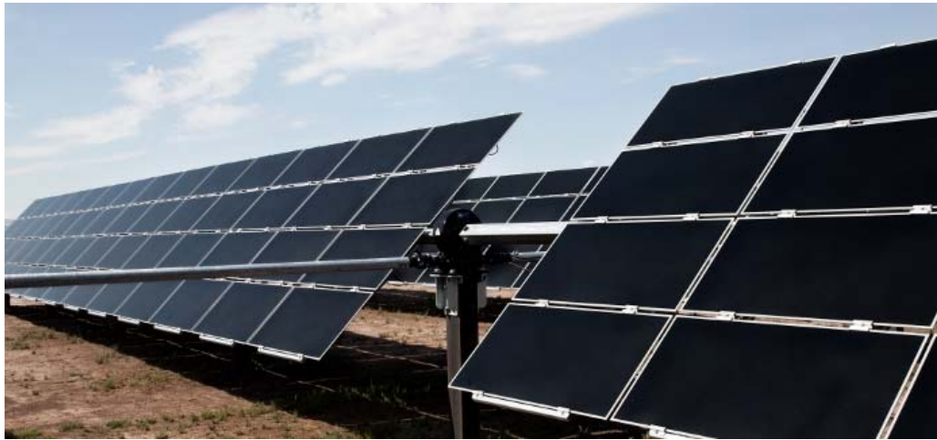
Plate 1. Example of a typical frameless solar array mounted on a single axis tracking system 10
