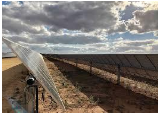
Fig 4 . Typical Solar Panel Arrangement
