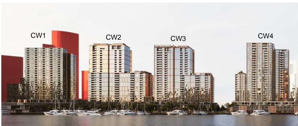
Figure 2: Approved and constructed developments to the east of the site.
