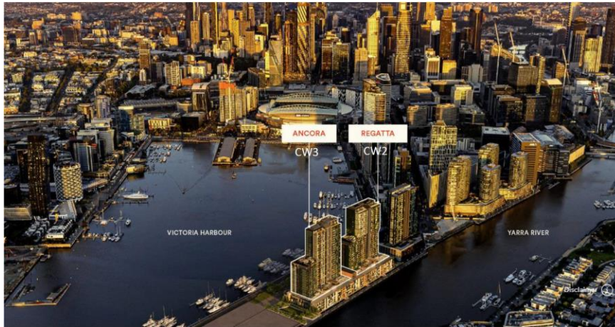
Figure 19: CW2 and CW3 looking east towards Collins Street
