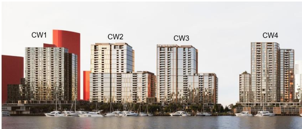
Figure 20: CW2, CW3 and CW4 looking south
