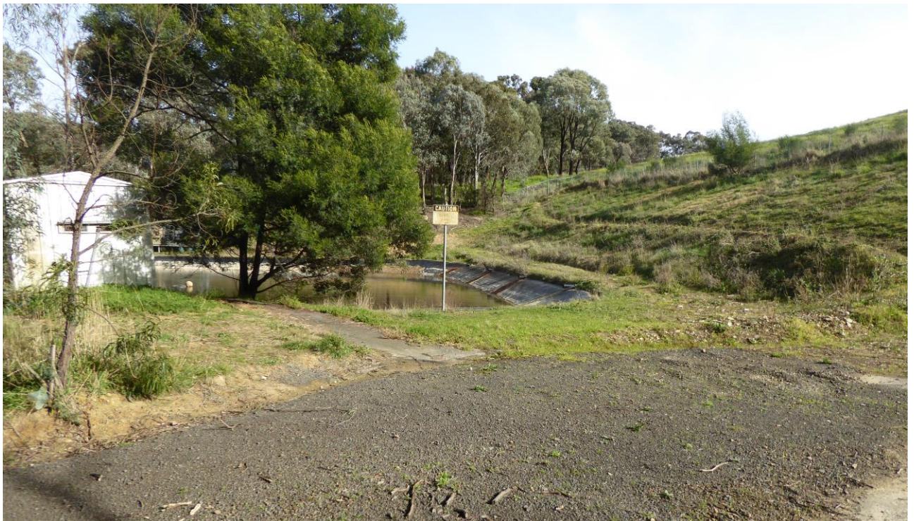
Figure 12 Existing dam in south-east corner of the site
