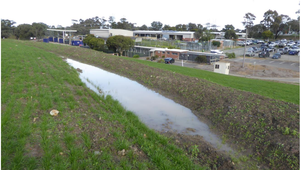
Figure 5 View south-east, showing the existing recycling facility, animal pound and associated structures
