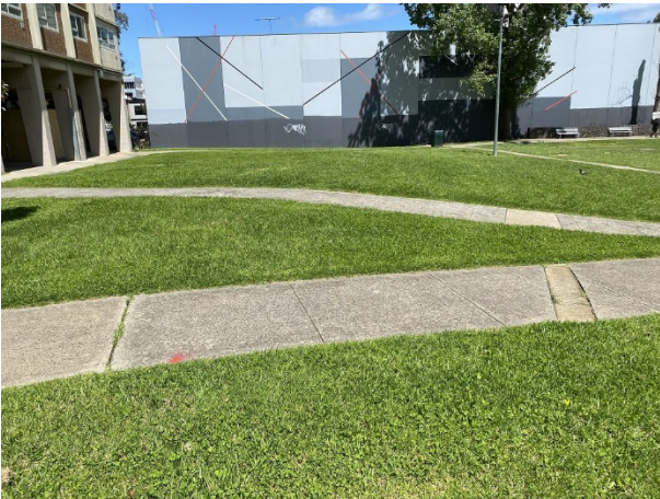
Above: Adjoining commercial zone presents windowless concrete panel walls to the common boundary
