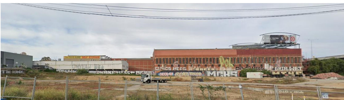
Figure 12 - View of southern interface.
