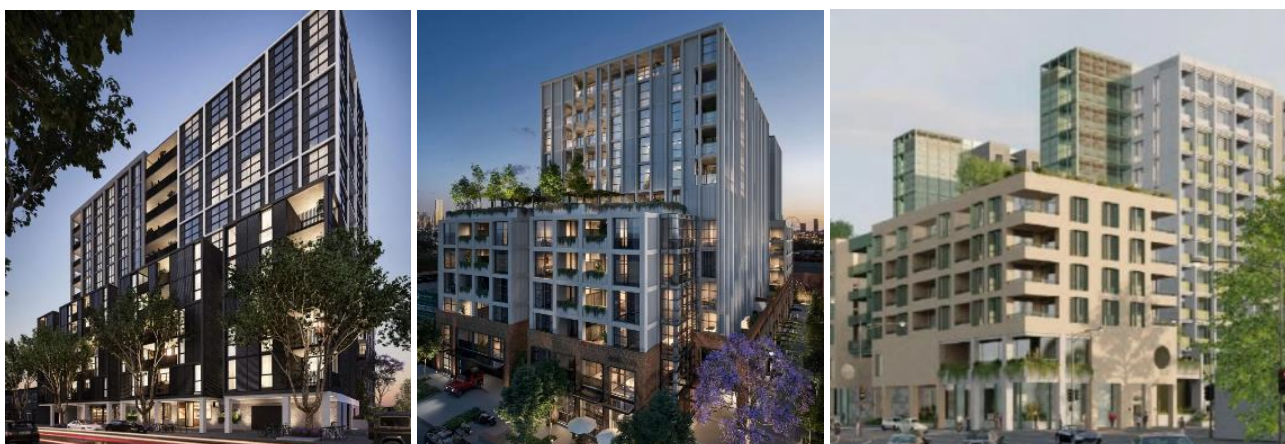
Figure 13 - L-R: Artists impressions of 139-149 Boundary Road, 77 Sutton Street, and 218-246 Macaulay Road & 23-35 Boundary Road.
