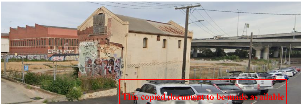
Figure 28 - View of Farrell's Stables building from Alfred Street
