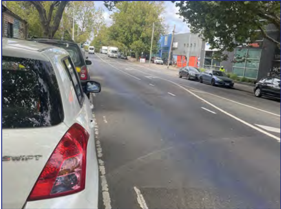
Figure 5: Boundary Road – View South
