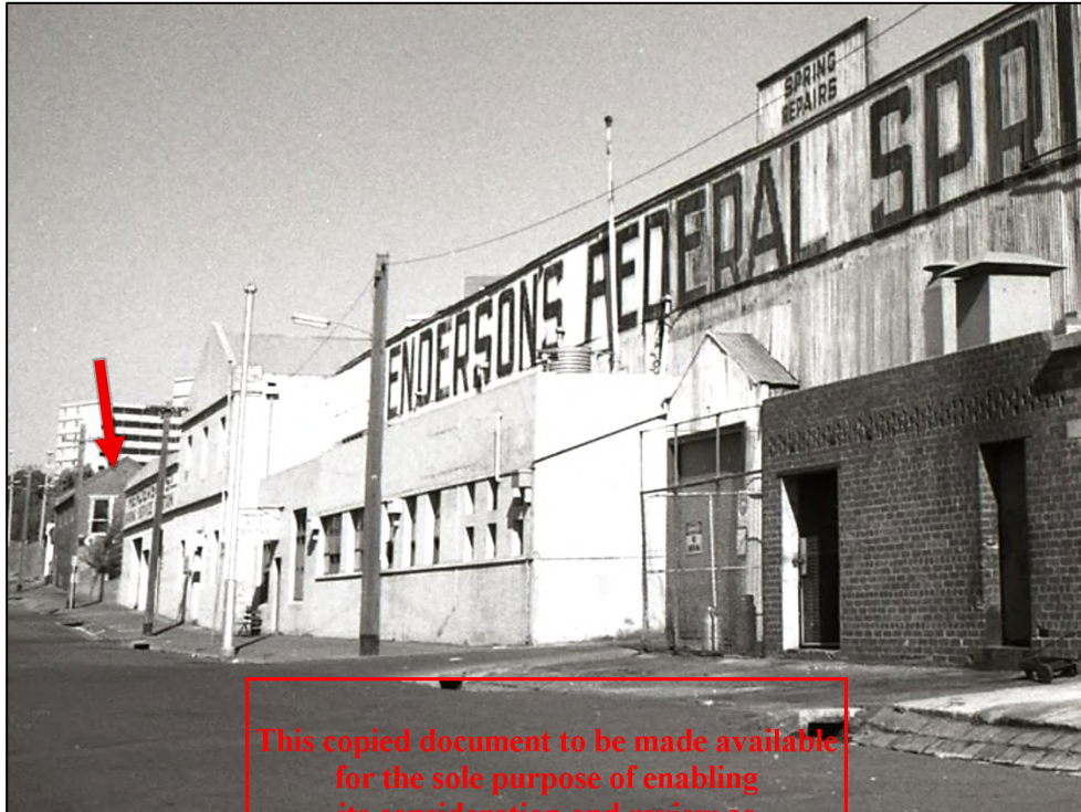
Figure 8 Another early 1980s view along the Hendersons Federal Spring Works Alfred Street frontage, with the stable visible at far left (denoted by the yellow arrow). Source: Graeme Butler, https://flic.kr/p/oWtsfE
