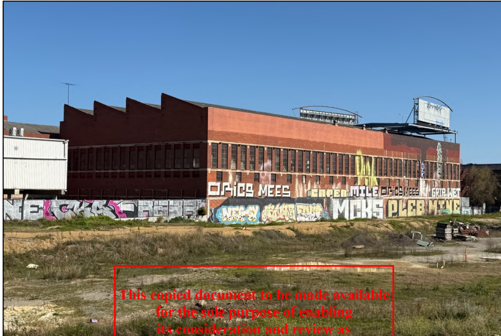
Figure 15 View of the rear from a high vantage point looking south across the subject site. Prior to the recent demolition of the industrial complex on the subject land, this elevation is understood to have been concealed from view.
