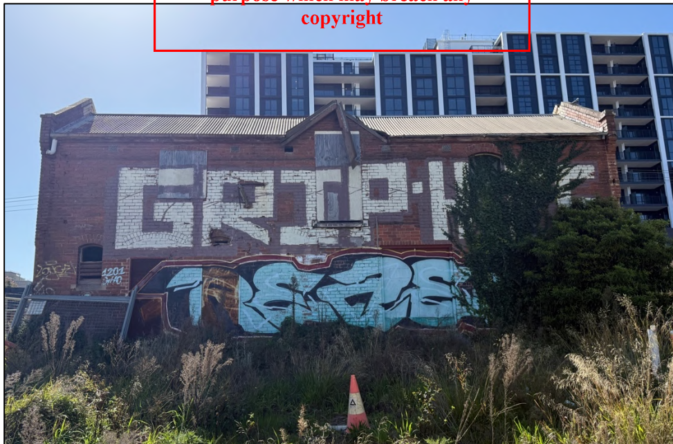
Figure 14 The rear south elevation faces into the site. The adjacent land is assumed to have originally been at grade but has since been excavated by demolition. The ground floor openings have been altered with the east side of building concealed by vegetation.
