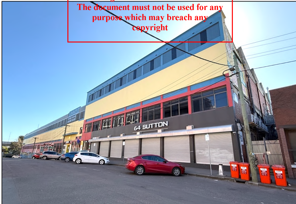
Figure 22 View of the extensive, multi-storey Sutton Street frontage of the Commonwealth Wool Store & Produce Company Ltd stores at 64-90 Sutton Street from further west along Sutton Street.
