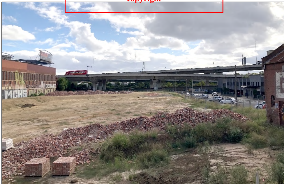
Figure 16 View west across the subject land, with the Moonee Ponds Creek Reserve and tollway overpass visible at centre. Partially visible at far left is the Commonwealth Wool Store & Produce Company Ltd stores at 64-90 Sutton Street and at far right, Farrell's Stables.
