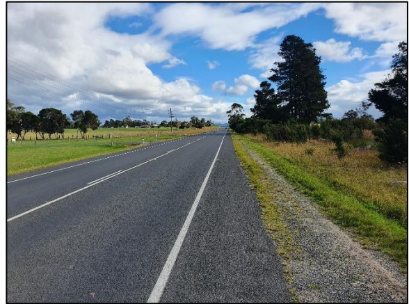
Figure 8: Firmins Lane – View West
