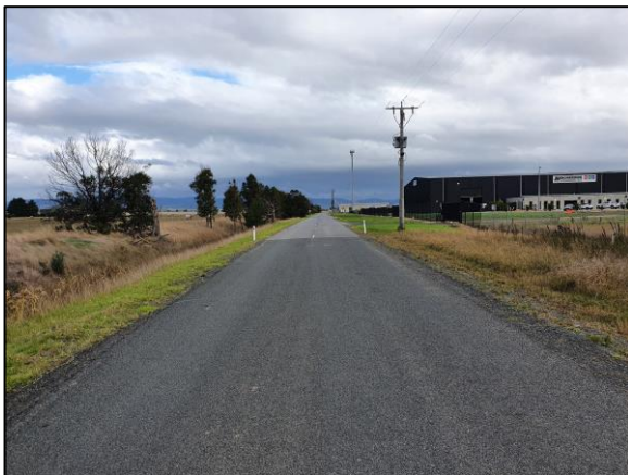
Figure 15: Groppi Road – View East
