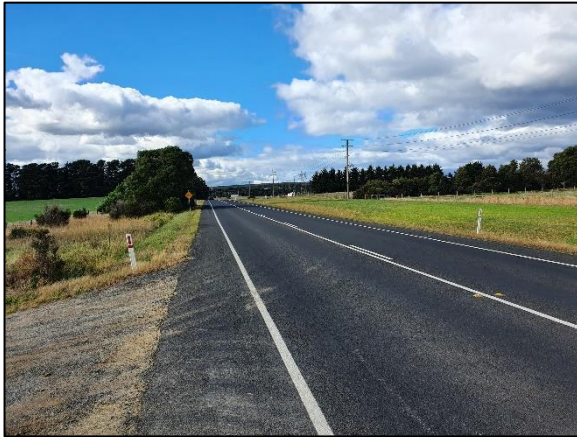
Figure 7: Firmins Lane – View East
