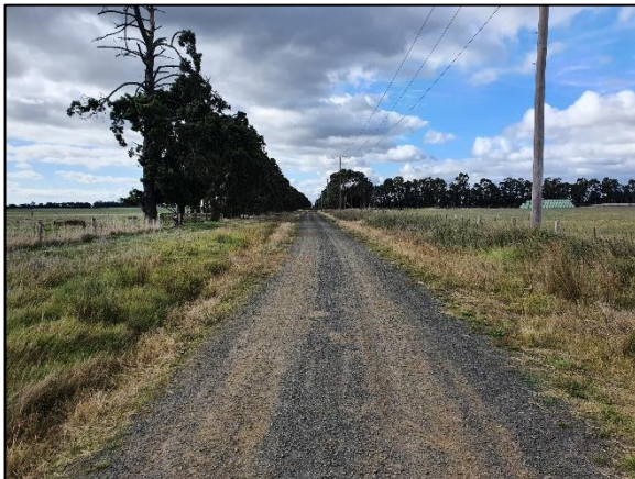
Figure 9: Walshs Road - View East
