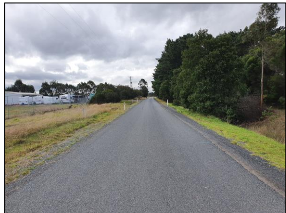
Figure 16: Groppi Road – View West
