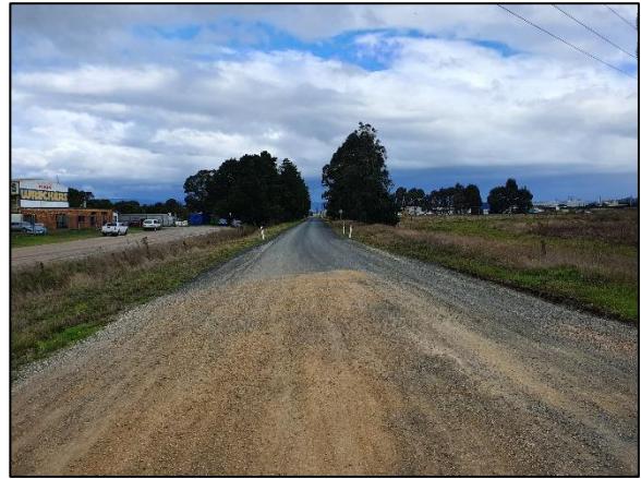
Figure 14: Buckleys Road – View South
