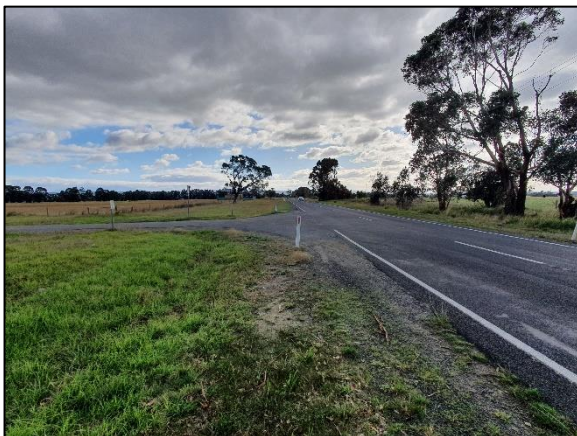
Figure 11: Hazelwood Road - View North
