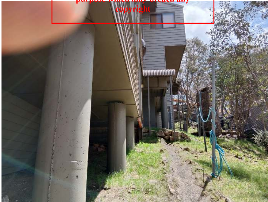
Plate 4. View looking northwest along the edge of the lodge
