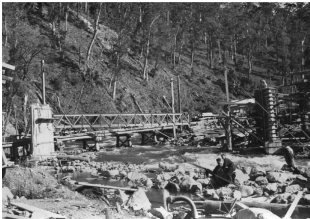
Figure 1 Construction of Clover Dam Power Station bridge, with the power station site to the right of the photograph and the piles for the bridge under construction (Photographs - SECV - Clover Power Station, 1940s)
