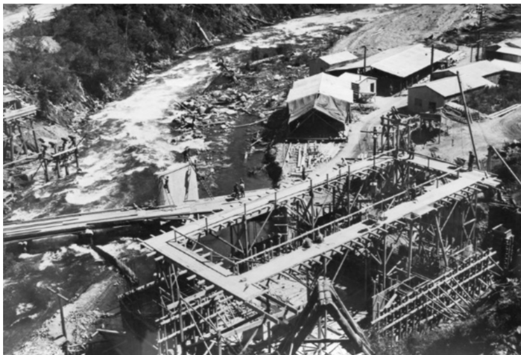
Figure 2 Construction of Clover Dam Power Station and bridge, with the power station site to in the foreground and the piles for the bridge under construction (Photographs - SECV - Clover Power Station, 1940s)
