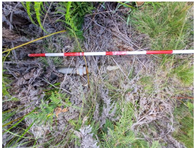
Photograph 24 Exposed section of pipe reported by AGL near the access track to Pole 553 (D. Carpenter, 14 February 2024)
