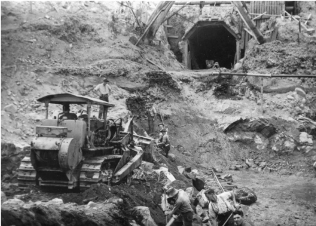
Figure 7 Image of combined manual and mechanical excavation occurring during the Kiewa Hydro Scheme construction (Photographs - SECV - Clover Power Station, 1940s)
