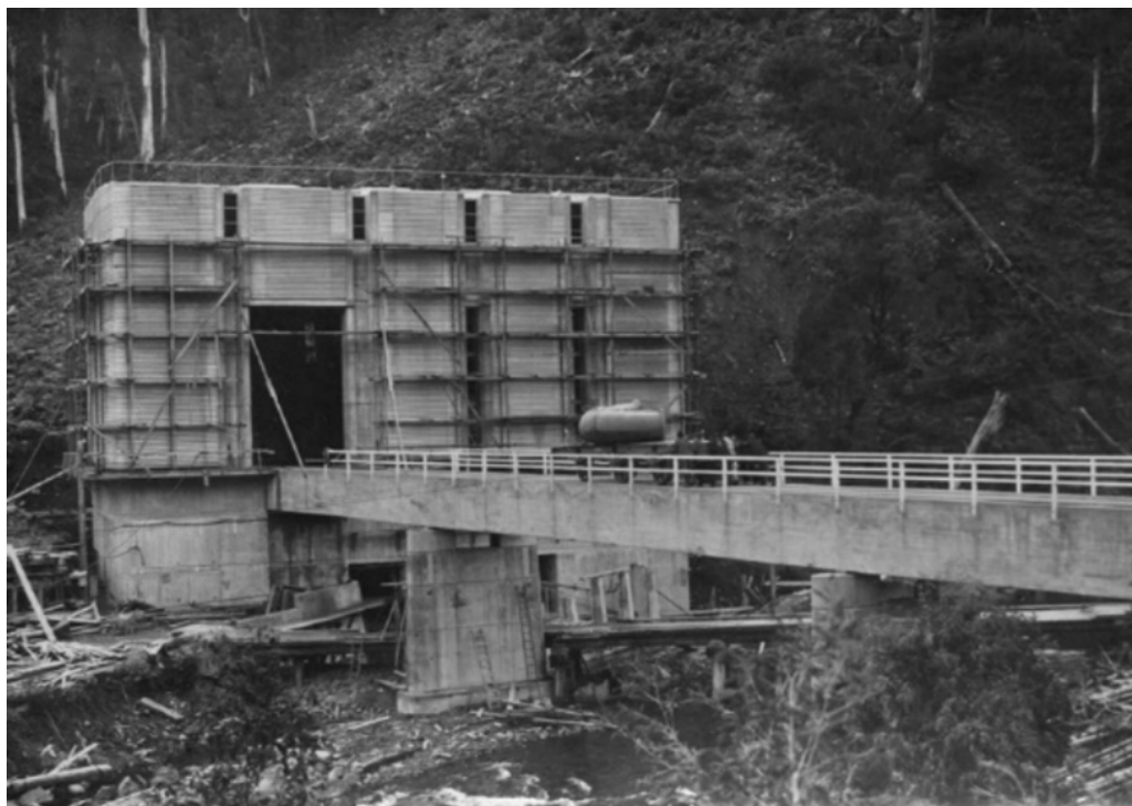
Figure 5 Clover Dam Power Station nearing completion, with the tail-bay location at the bottom of the photograph (Photographs - SECV - Clover Power Station, 1940s)
