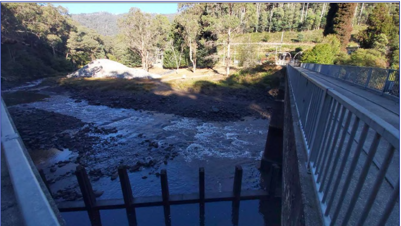
Picture 4 View across existing Tail Bay from Power Station
