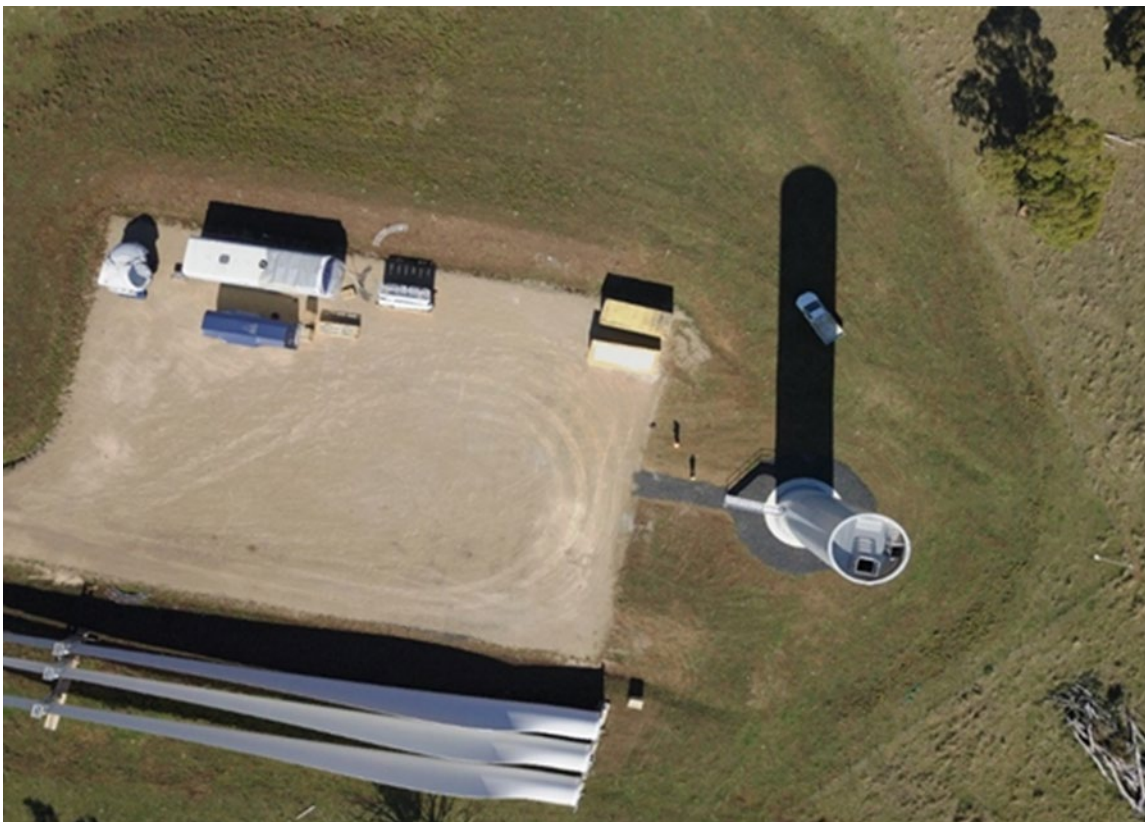
Photo 3.4 Hardstand, Tower Foundation and Blade Laydown Area at Sapphire Wind Farm
