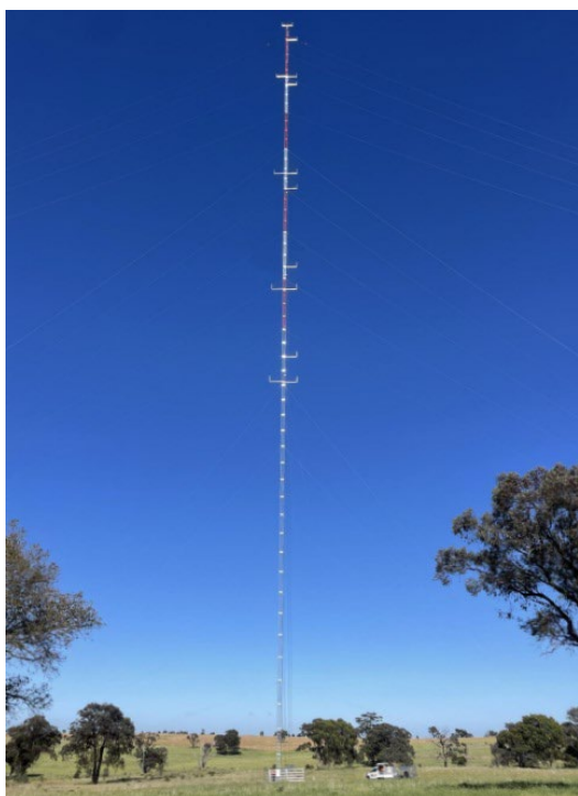
Photo 3.10 Example of a wind monitoring mast
