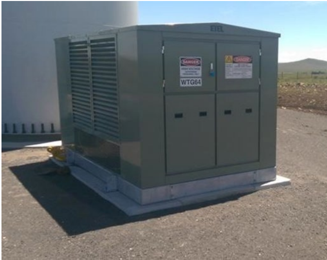
Photo 3.8 Example of a Generator Transformer Located Outside of the Tower at Boco Rock Wind Farm
