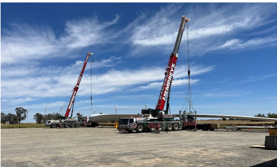
Photo 3.7 A Blade Being Installed at Murra Warra Wind Farm
