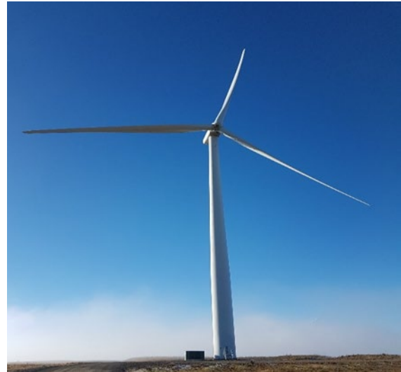
Photo 3.8 Example of a Generator Transformer Located Outside of the Tower at Boco Rock Wind Farm
