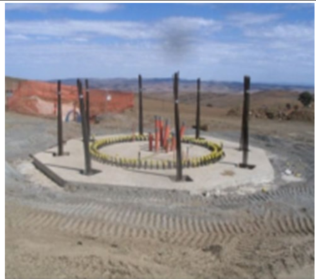
Photo 3.3 WTG foundation type: rock anchor
