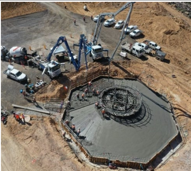
Photo 3.2 WTG foundation type: gravity
