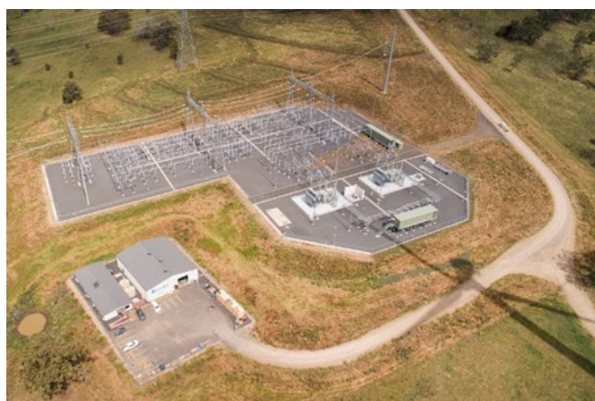
Photo 3.9 Example of an O&M Compound (foreground) Shown in Front of the Substation at Sapphire Wind Farm, NSW
