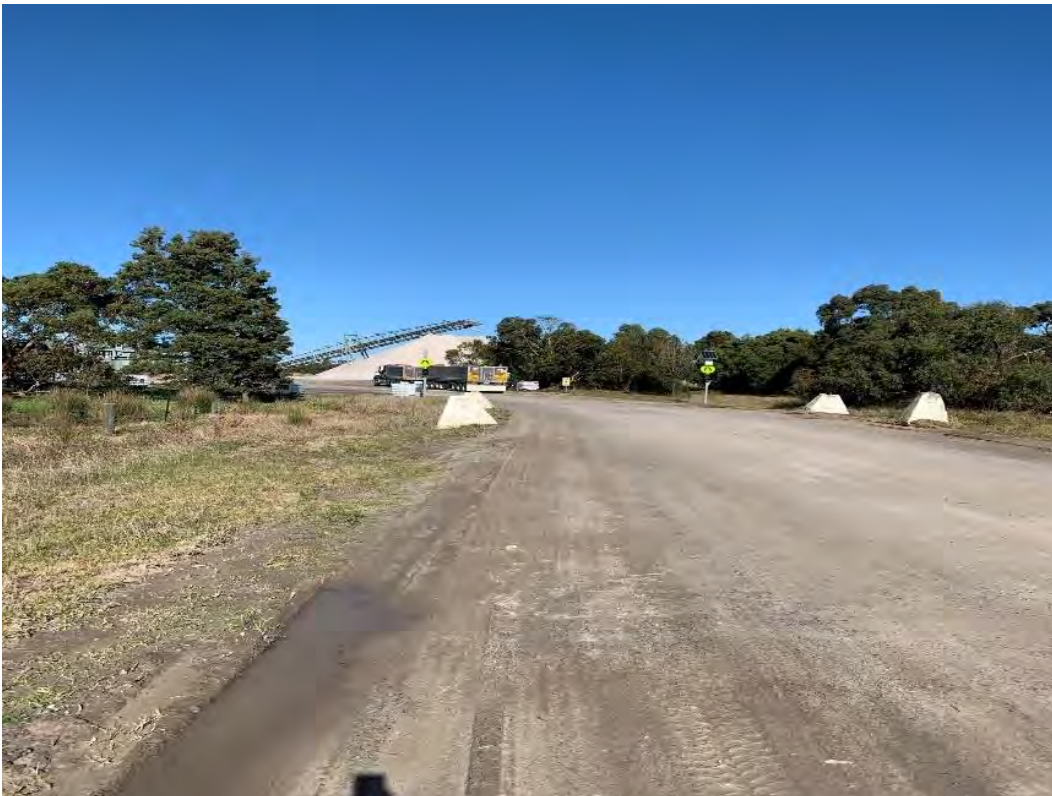
Figure 3.15: Access Road crossing at Reach B
