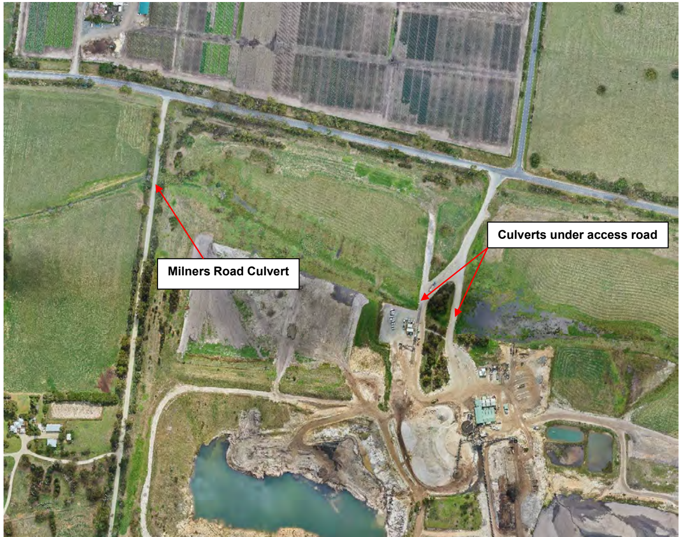
Figure 2-5: Existing Culvert Crossing Locations
