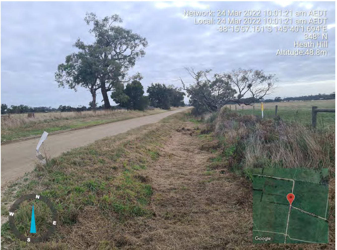
Figure 4-5: Channel along Pooles Road
