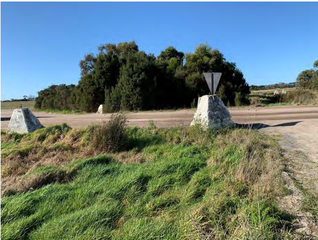
Figure 3.17: Access Road crossing channel upstream at Reach B
