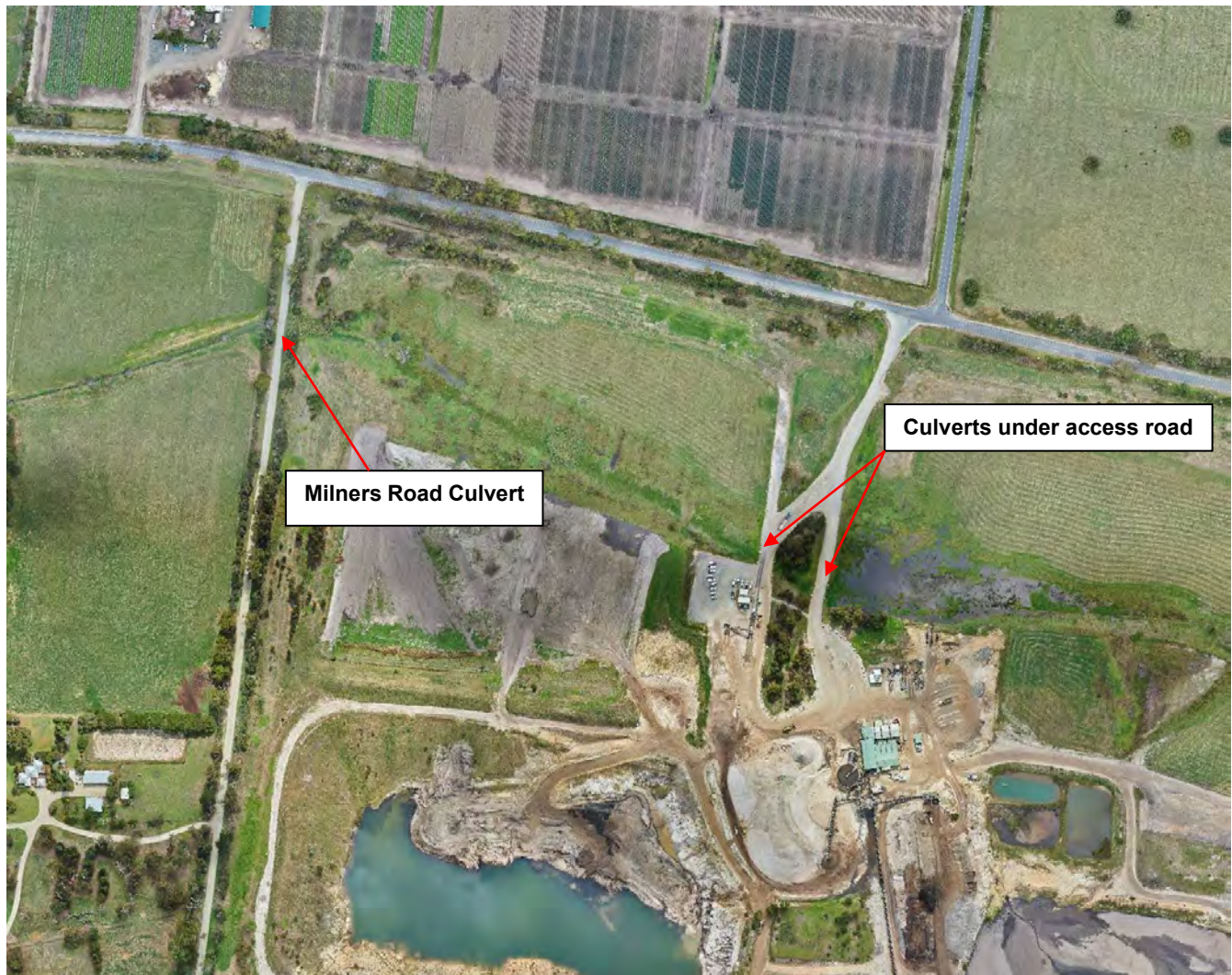
Figure 2-5: Existing Culvert Crossing Locations
