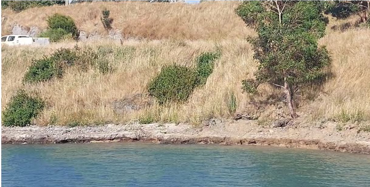
WEST PIT WESTERN BATTER - FACING SOUTHWEST - 11/01/2023
