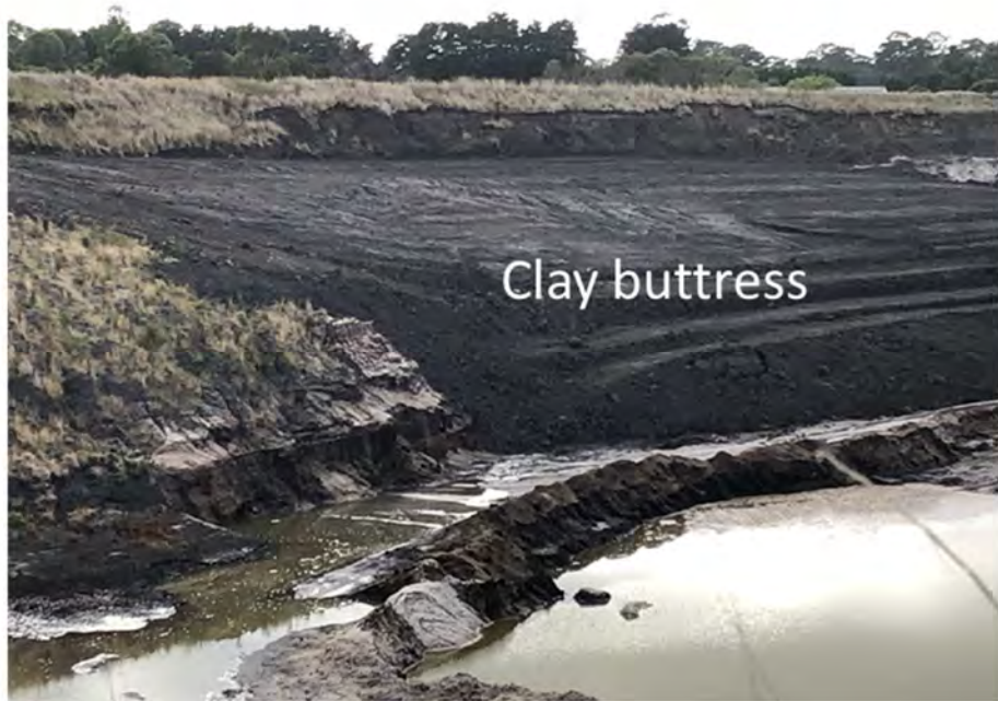
Temporary clay buttress on the north side of the east pit
