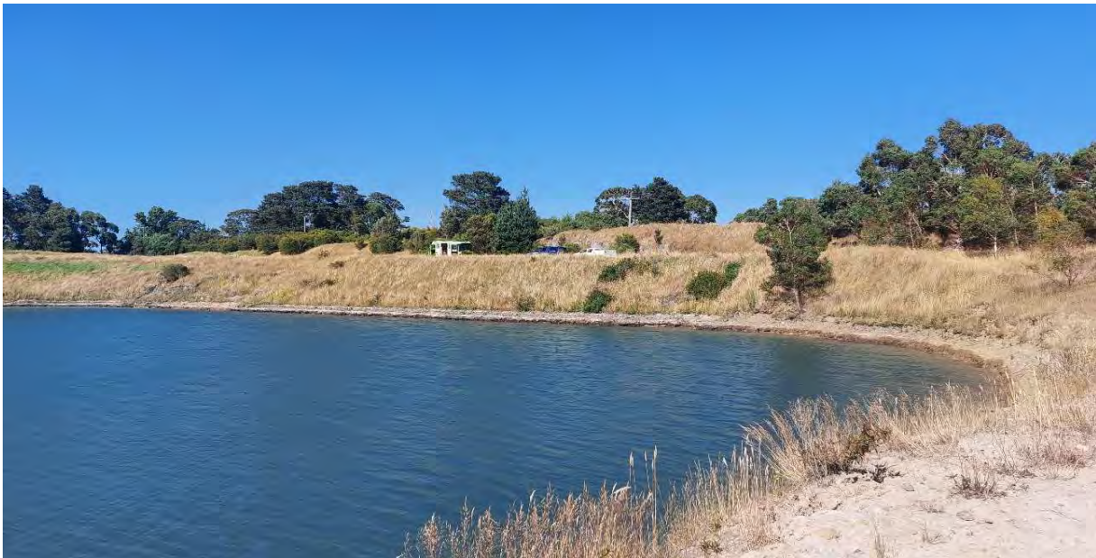
WEST PIT WESTERN BATTER - FACING SOUTHWEST - 11/01/2023
