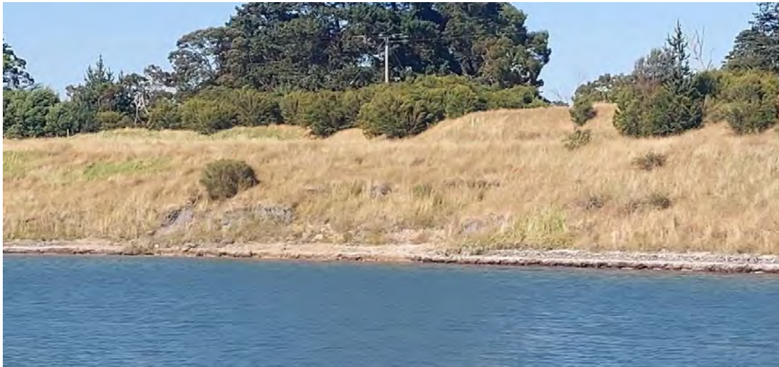
Figure 20: Grass cover on batters of the west pit (facing southwest 11 January 2023)
