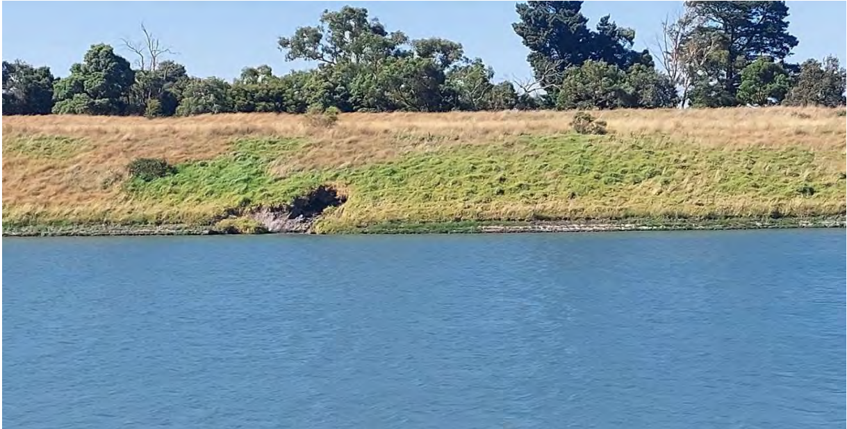
WEST PIT SOUTHERN BATTER - FACING SOUTH - 11/01/2023
