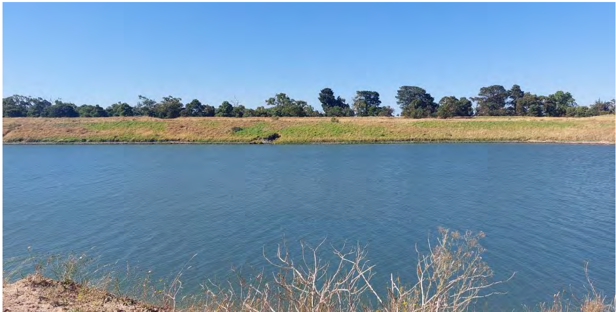
WEST PIT SOUTHERN BATTER - FACING SOUTH - 11/01/2023
