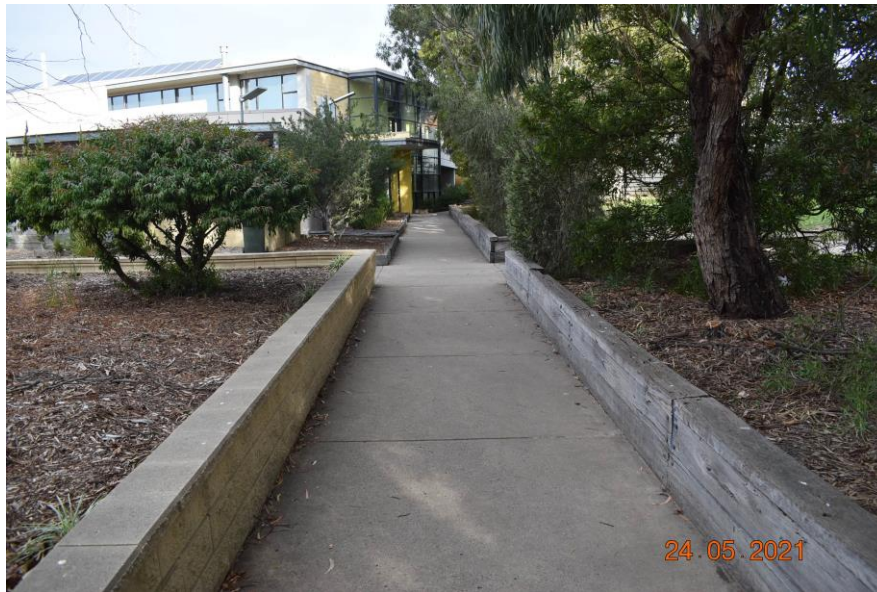
Figure 2: Looking south at the Loyola Administration building with trees and shrubs growing in raised garden beds
