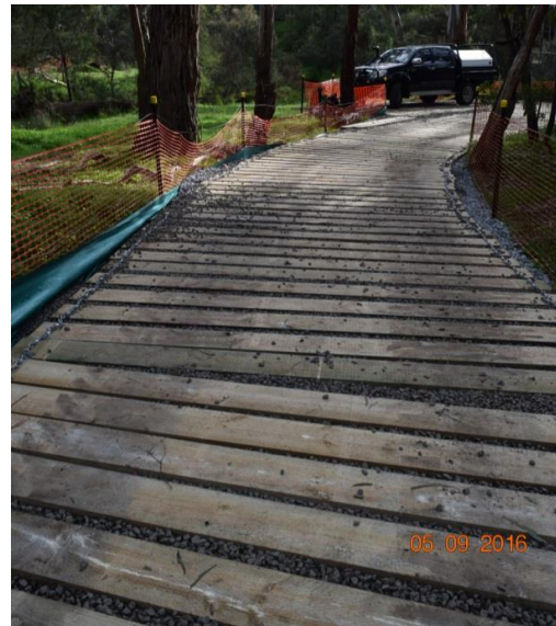
Figure 10: Rumble boards over crushed rock.
