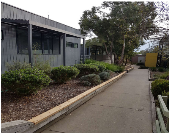
5 The Existing Loyola Administration Centre to be removed/demolished by the school. Extent of removal to be confirmed.
