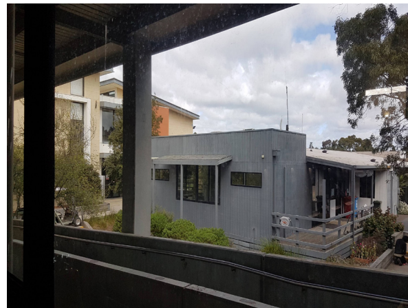
6 View from the Information Learning Centre (ILC) of the Existing Loyola Administration Centre to be removed/demolished by the school.
