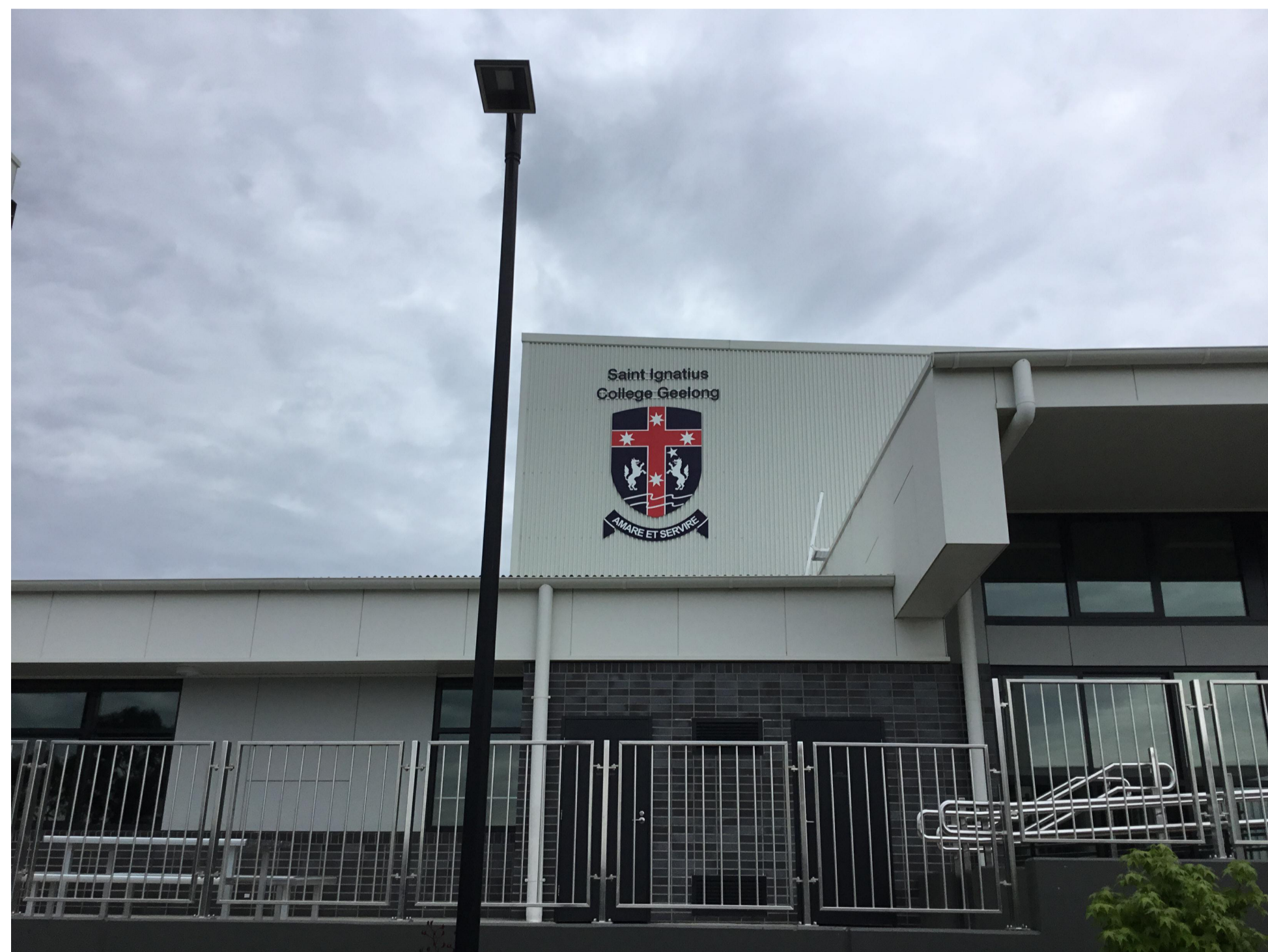
EXISTING FRONT SIGNAGE 1 - PENINSULA DRIVE DIMENSIONS: 2.5m(W) x 3.7m(H) HEIGHT ABOVE NGL: 6.5m ILLUMINATED: NO HOURS: N/A BAFFLE PROVIDED: NO
