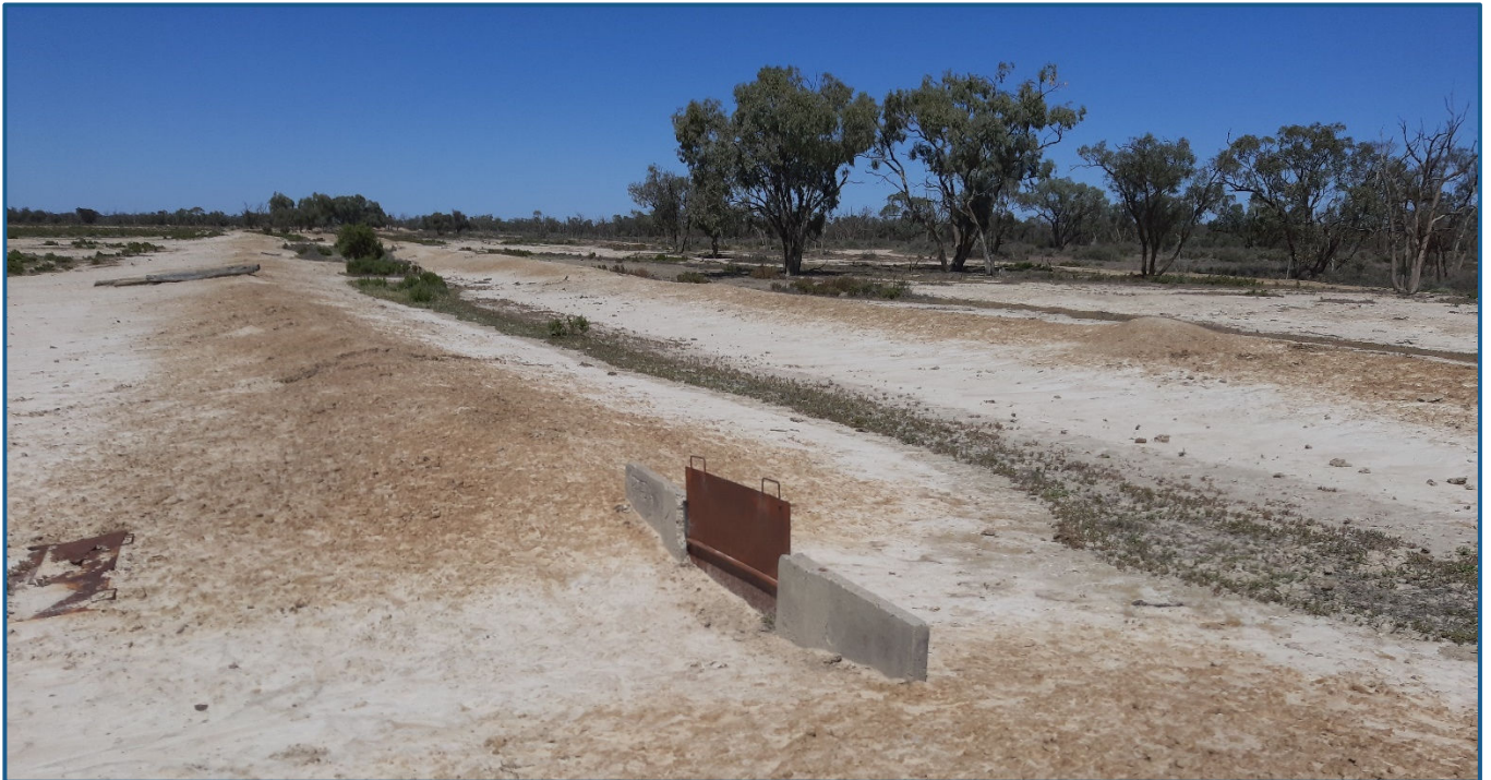
Image 4: An unmaintained and now-defunct earthen irrigation water supply channel and outlet in the southwest of the site.
