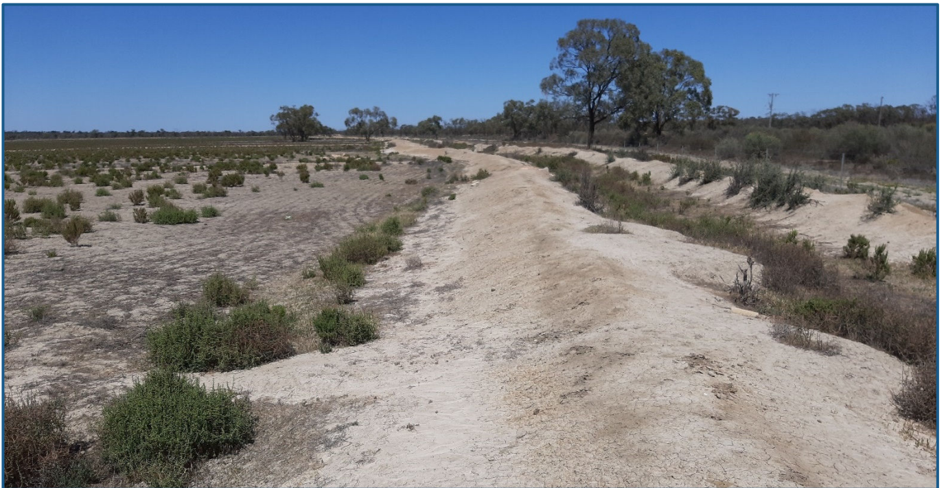
Image 5: An unmaintained and now-defunct earthen irrigation water supply channel is located along the western boundary of the site.
