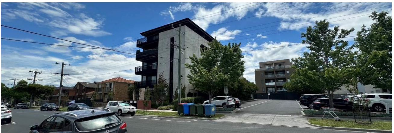
Figure 17 – 6 Hemmings Street, Dandenong (200 metres west of the subject site)
