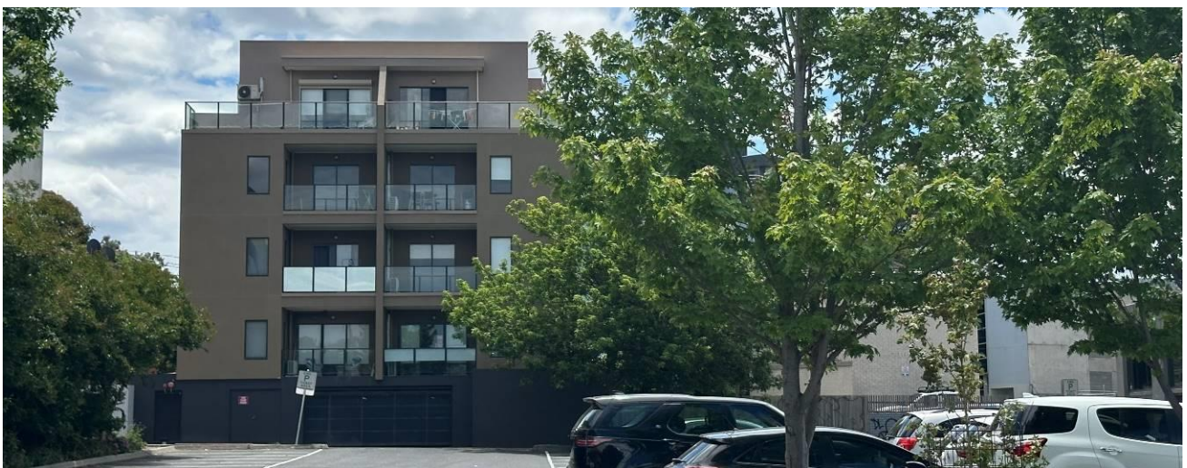
Figure 18 – 3 Close Avenue, Dandenong (200 metres west of the subject site)
