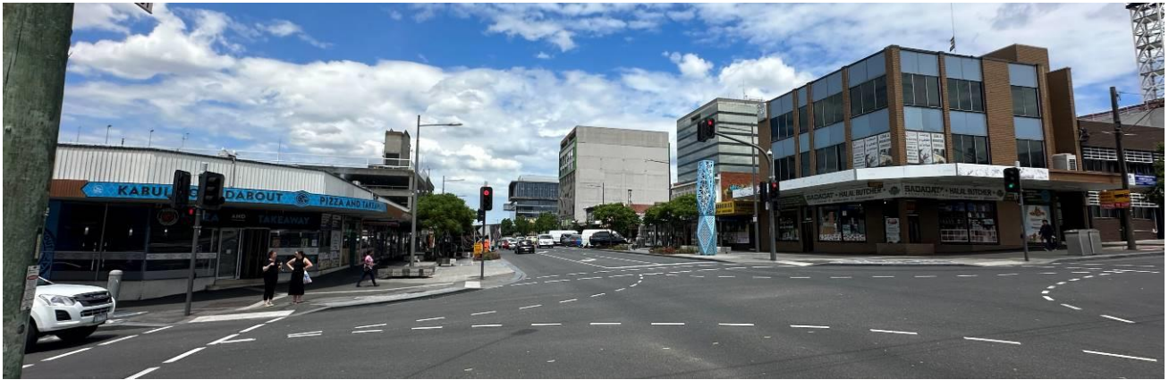
Figure 16 – Looking south along Thomas Street through the civic centre core
