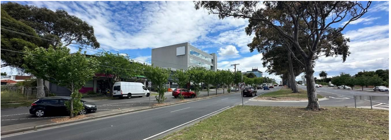
Figure 11 – Looking northwest along Princes Highway towards the commercial buildings
