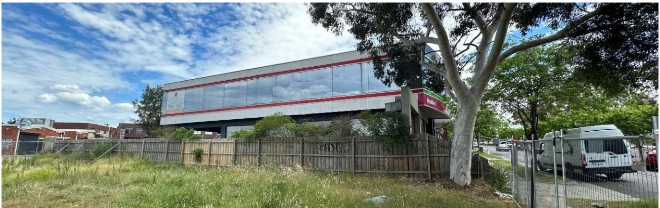
Figure 9 – 29 Princes Highway interface with the subject site
