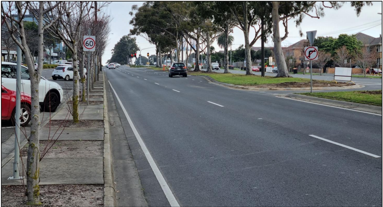
Figure 5 Princes Highway facing north from adjacent to the subject site
