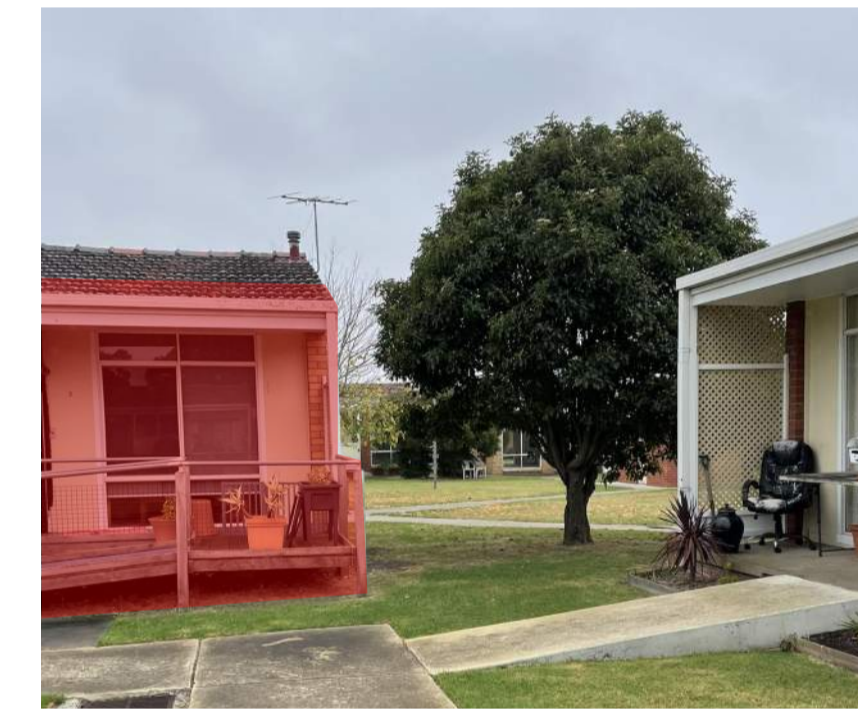
VIEW 06: EXISTING ILU (PARTIAL DEMOLITION)
