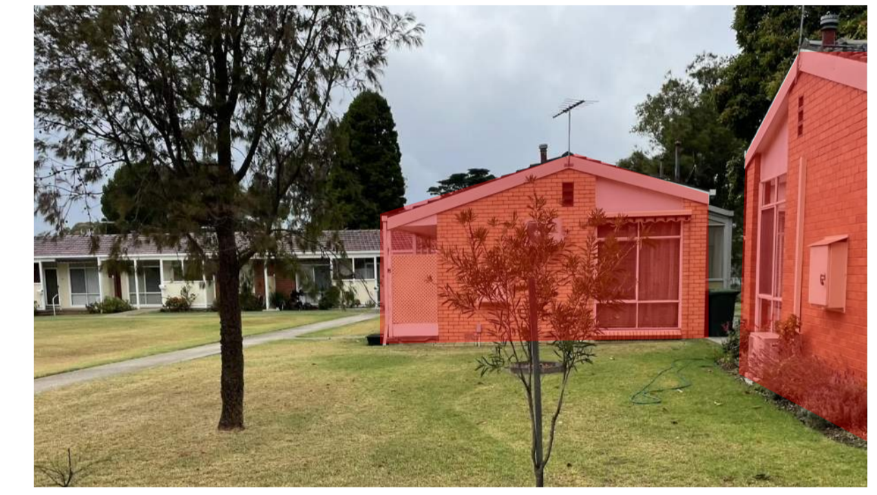
VIEW 03: EXISTING ILU'S TO BE DEMOLISHED (LOOKING EAST)
