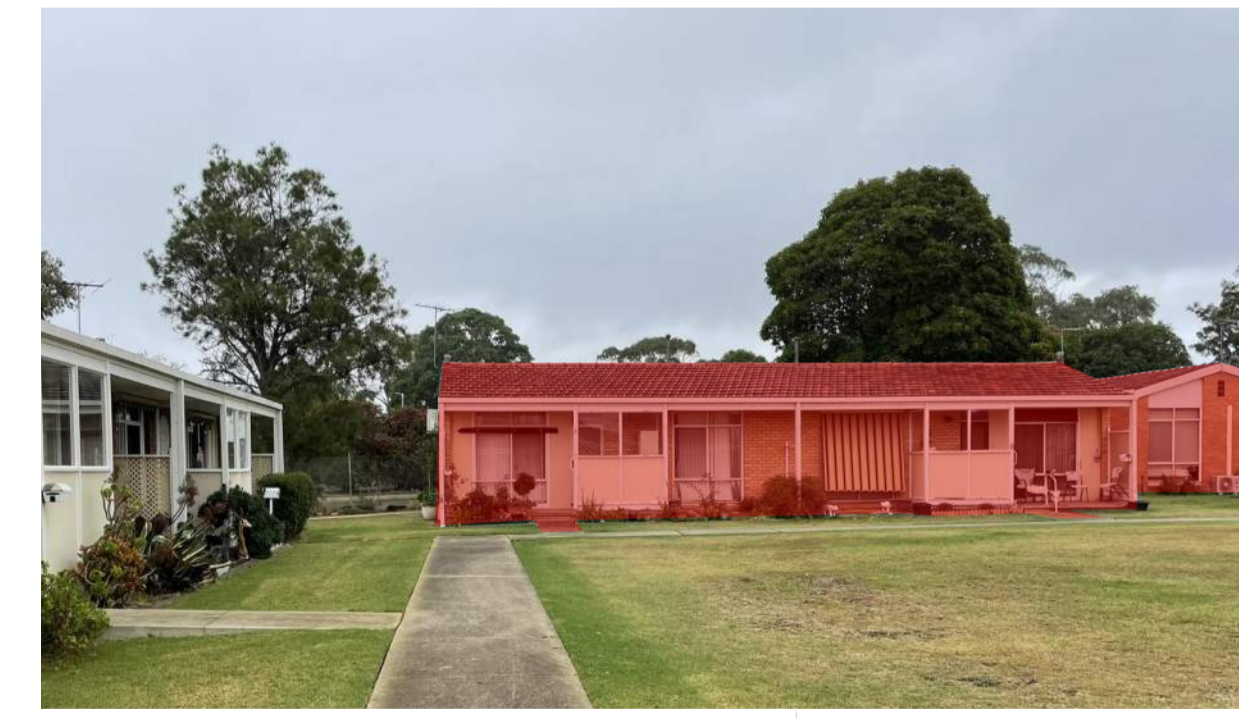
VIEW 07: EXISTING ILU'S TO BE DEMOLISHED (LOOKING SOUTH)
