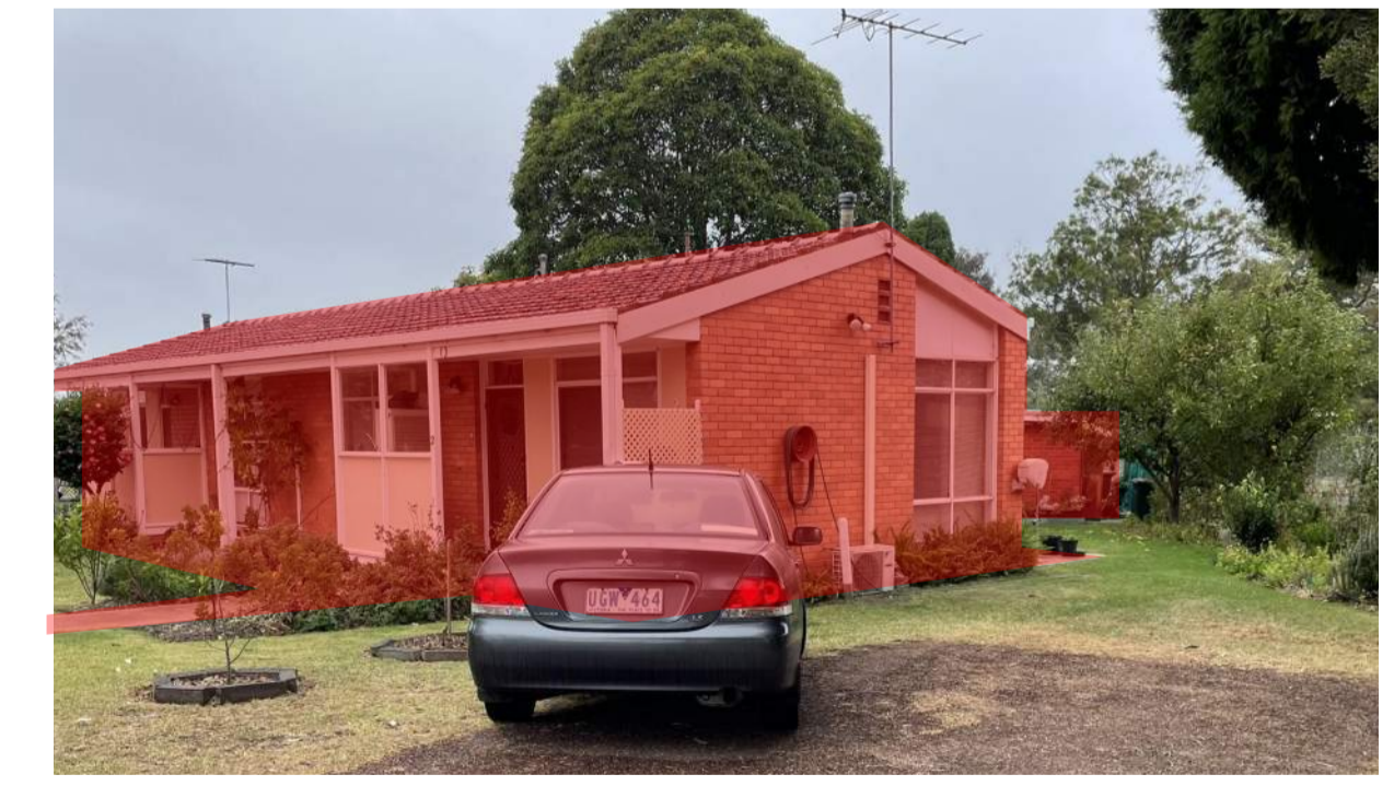
VIEW 04: EXISTING ILU'S TO BE DEMOLISHED (LOOKING EAST)
