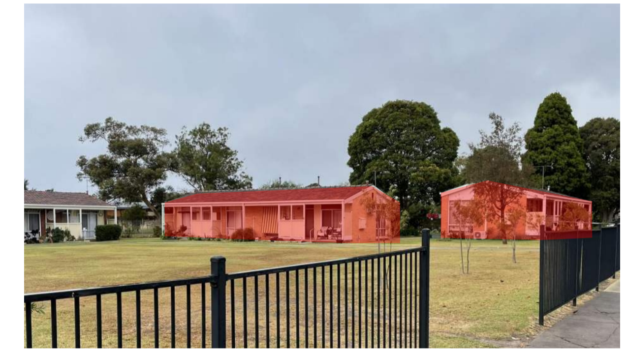
VIEW 02: EXISTING ILU'S TO BE DEMOLISHED (LOOKING SOUTH)
