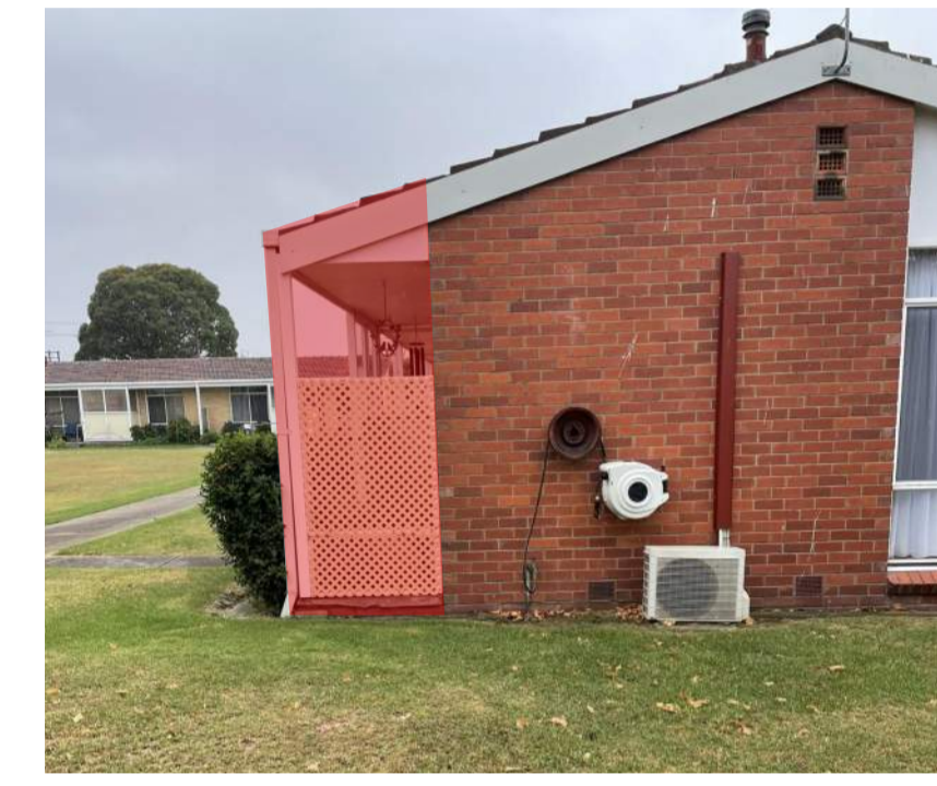
VIEW 05: EXISTING ILU (PARTIAL DEMOLITION)
