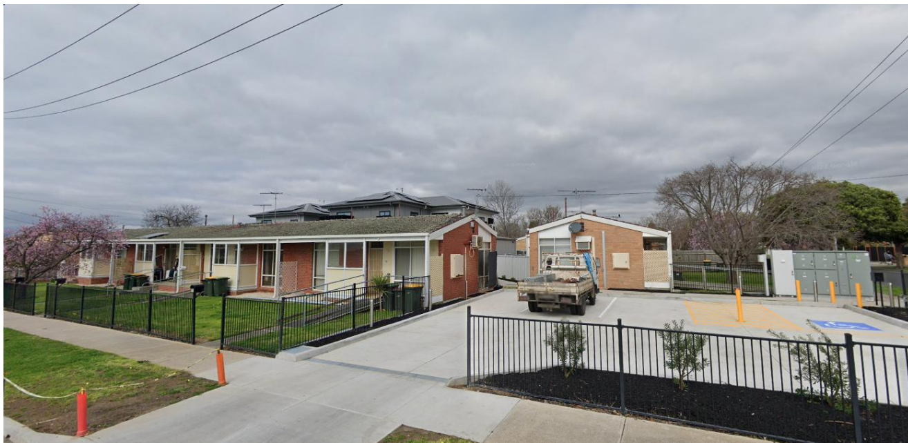
Figure 4 – 24 McClelland Street as viewed from the intersection of McClelland Street and Vistula Avenue looking south-east
