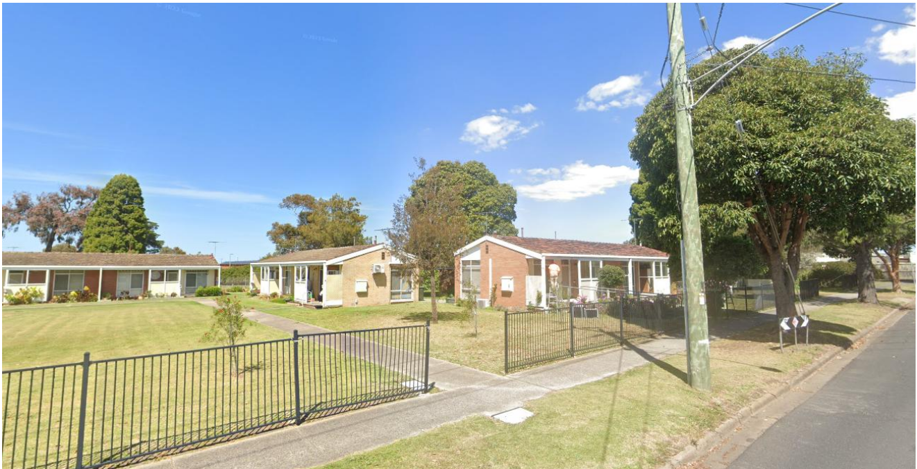
Figure 2 – The Site and the area of works, viewed from McClelland Street looking south-east
