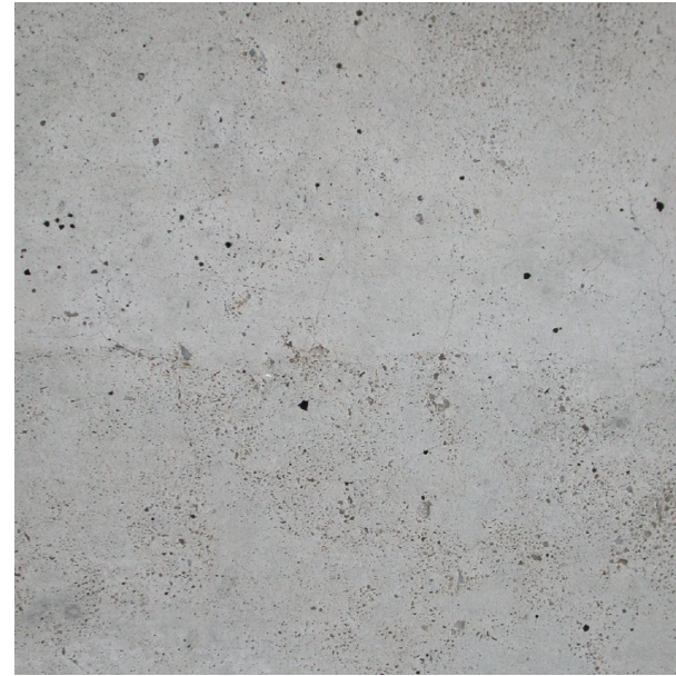
C1_CONCRETE FINISH WALLS & FLOORING
