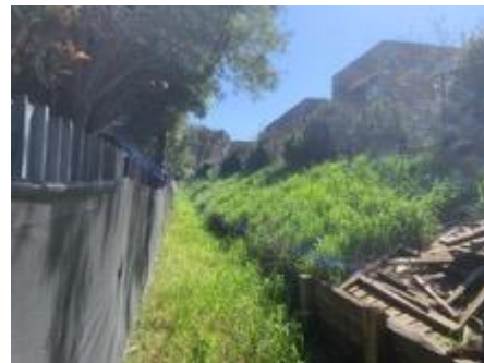
Image 13.16 – Area adjacent to proposed bus drop off / pickup. Notice difference in elevation from privately owned trees to existing roadway
