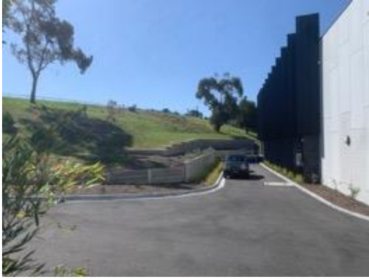
Image 13.17 – Retaining wall site adjacent to football oval
