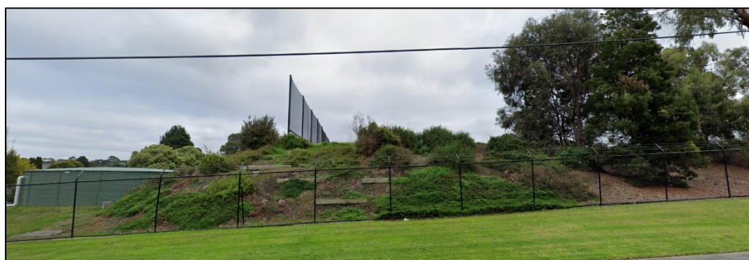
Figure 3: Google Streetview image showing the existing conditions of the southern east corner of Stanley Road
