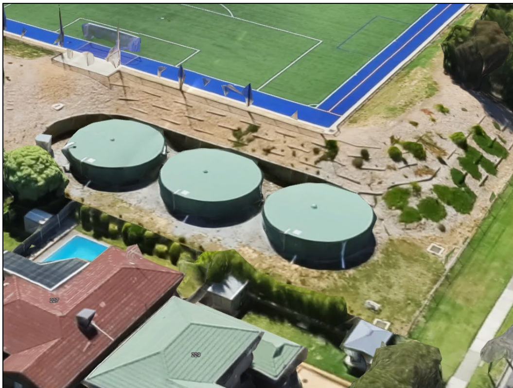
Figure 2: Google Earth photo showing the existing retaining wall and level changes throughout the south of the site.
