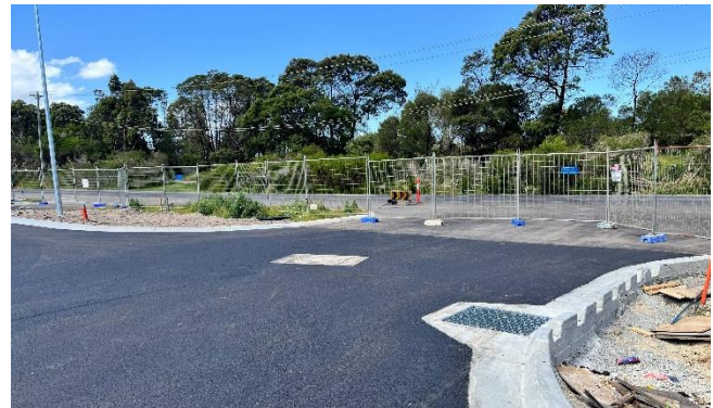
Figure 13 New main site entry from Pearcedale Road (facing towards the east)
