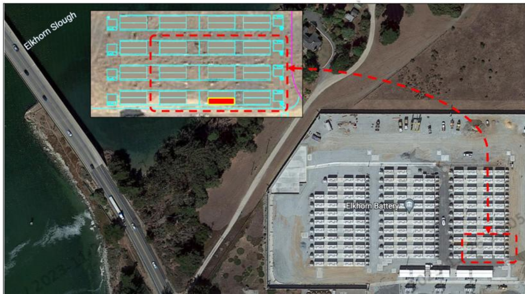
Figure 18: Overview of Elkhorn BESS and Megapack on fire.
