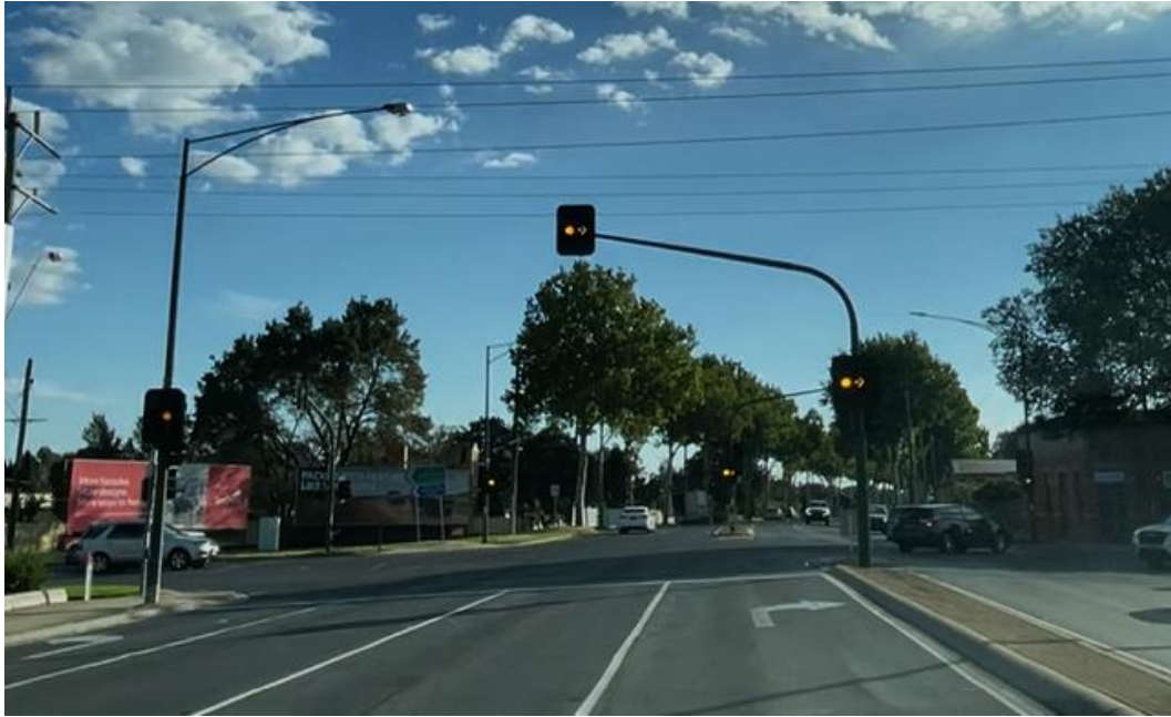
FIGURE 9: HIGH STREET / OAK STREET INTERSECTION – SOUTH APPROACH
