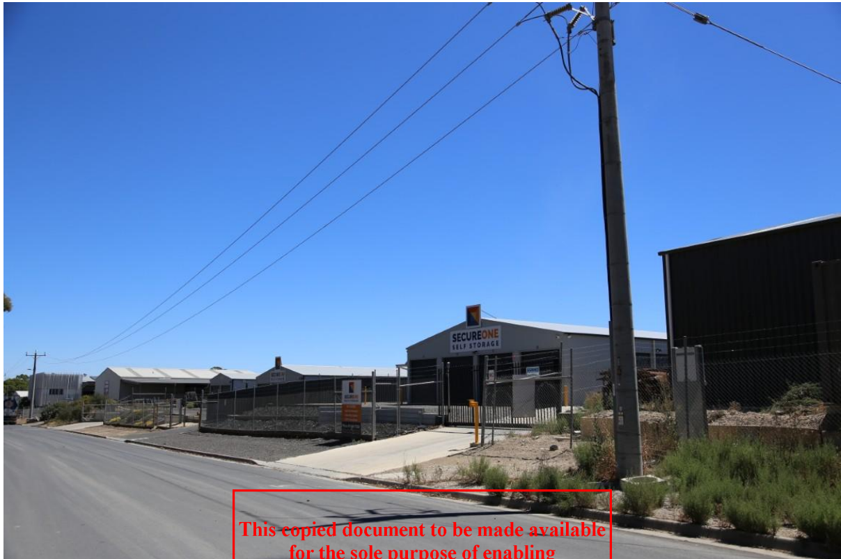
Figure 21 – Industrial facilities are located to the west of the Project area, north of Gray Street and between Coonooer Street and Allingham Street.
