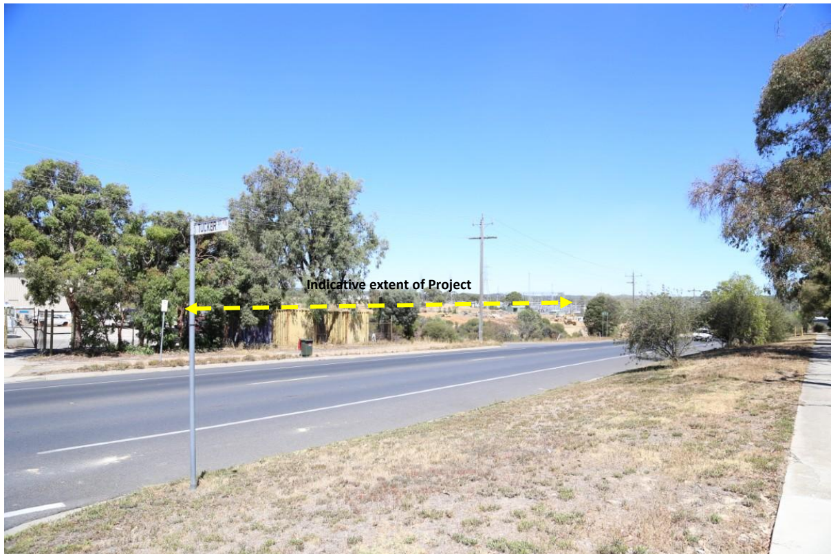
Figure 51 – VP1 –Existing view southwest towards the Project area from Hattam Road.
