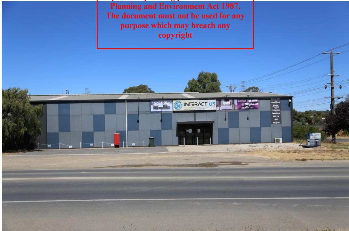
Figure 35 - Industrial building to the northwest of the Project site at the corner of Hattam Street and Allingham Street.
