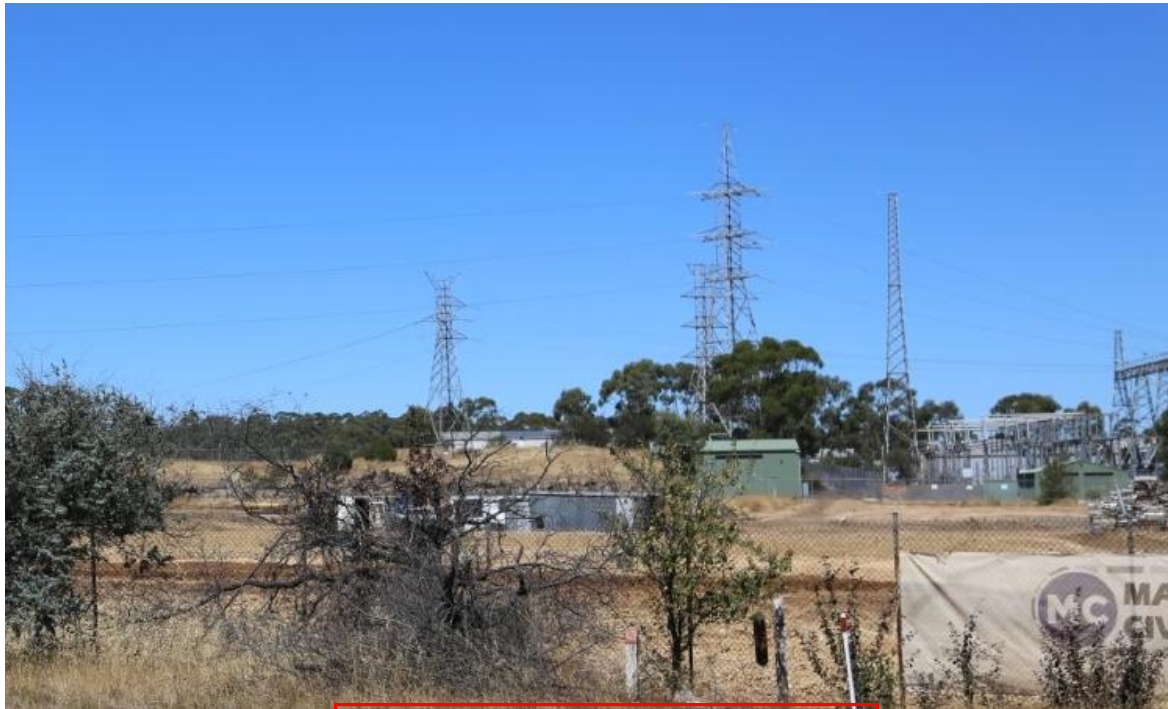
Figure 15 – An existing HV Powerline traverses the landscape to the southwest of the Project area.
