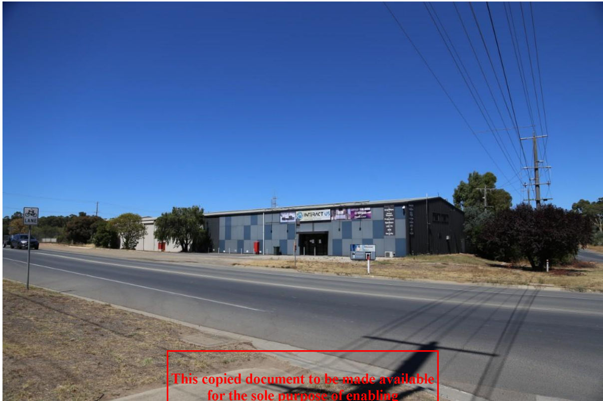
Figure 19 - Industrial facility to the northwest of the Project area at the corner of Hattam Street and Allingham Street.
