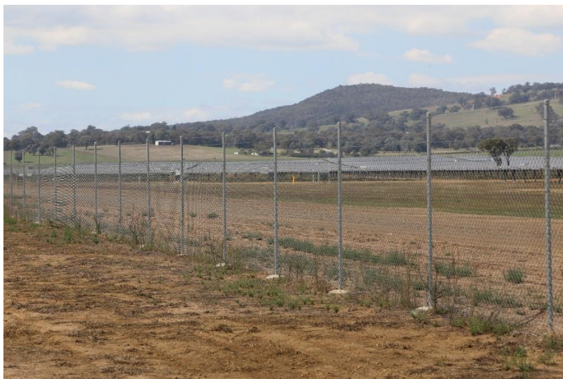
Figure 10 – Typical security fence.
