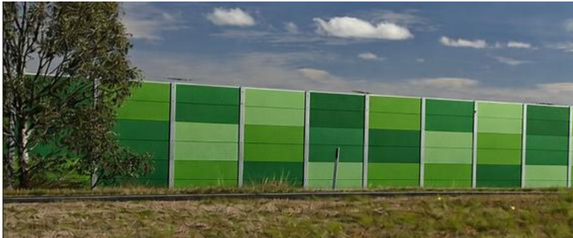
Figure 9 - Example of acoustic wall.
