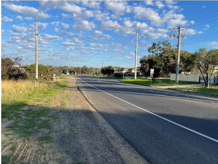
FIGURE 5: HATTAM STREET FACING WEST
