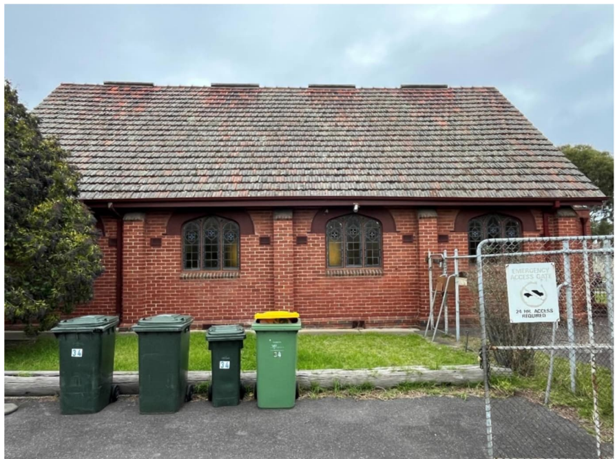
Figure 3: North elevation of former church on the subject site
