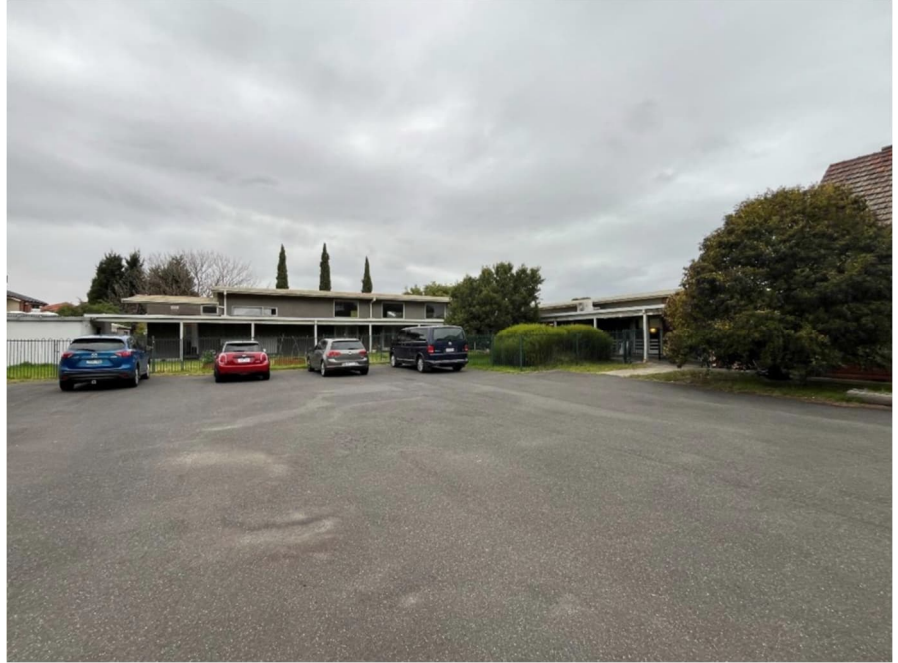
Figure 4: Existing 'L' shaped building on the subject site
