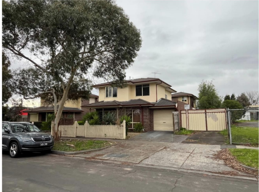
Figure 6: 36-38 George Street, north of the subject site
