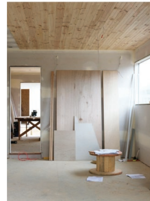
Shand Road project, recently completed
