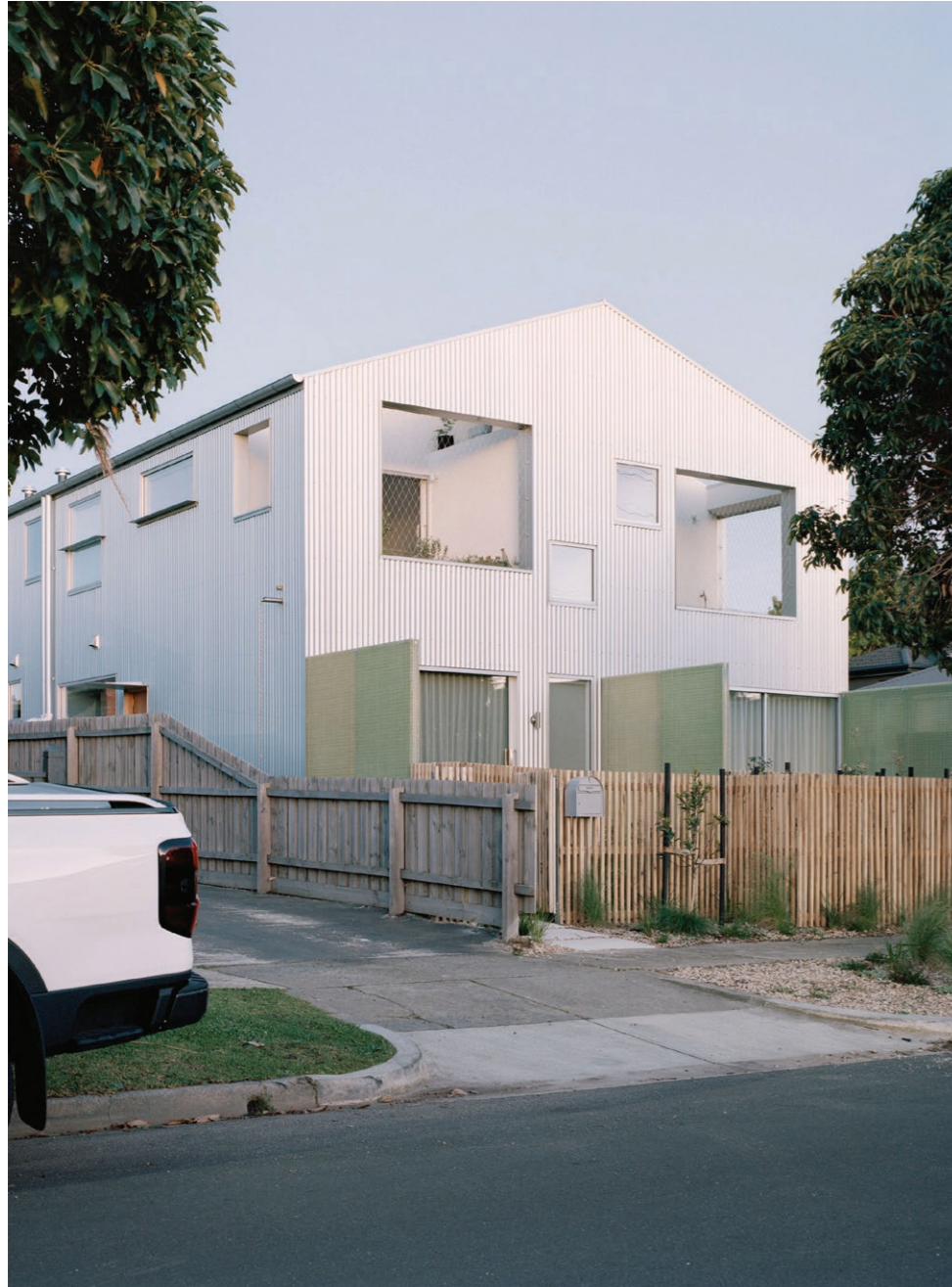
Shand Road project, recently completed
