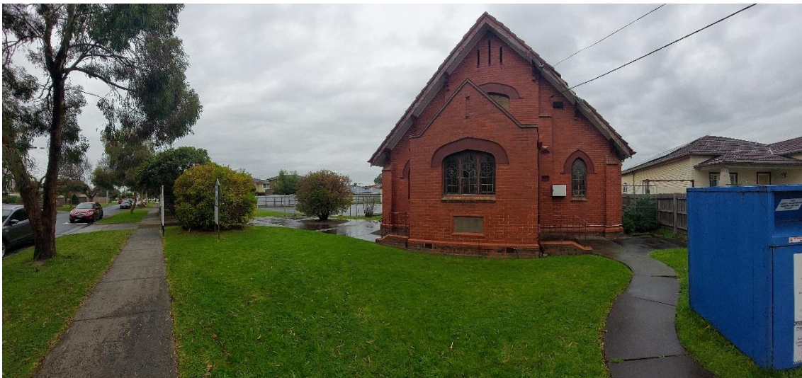
Plate 1: Panoramic view of the front of the site.
