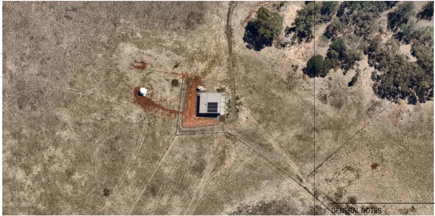
EXISTING SCHOOL BUILDING - OBSERVATION CENTRE
