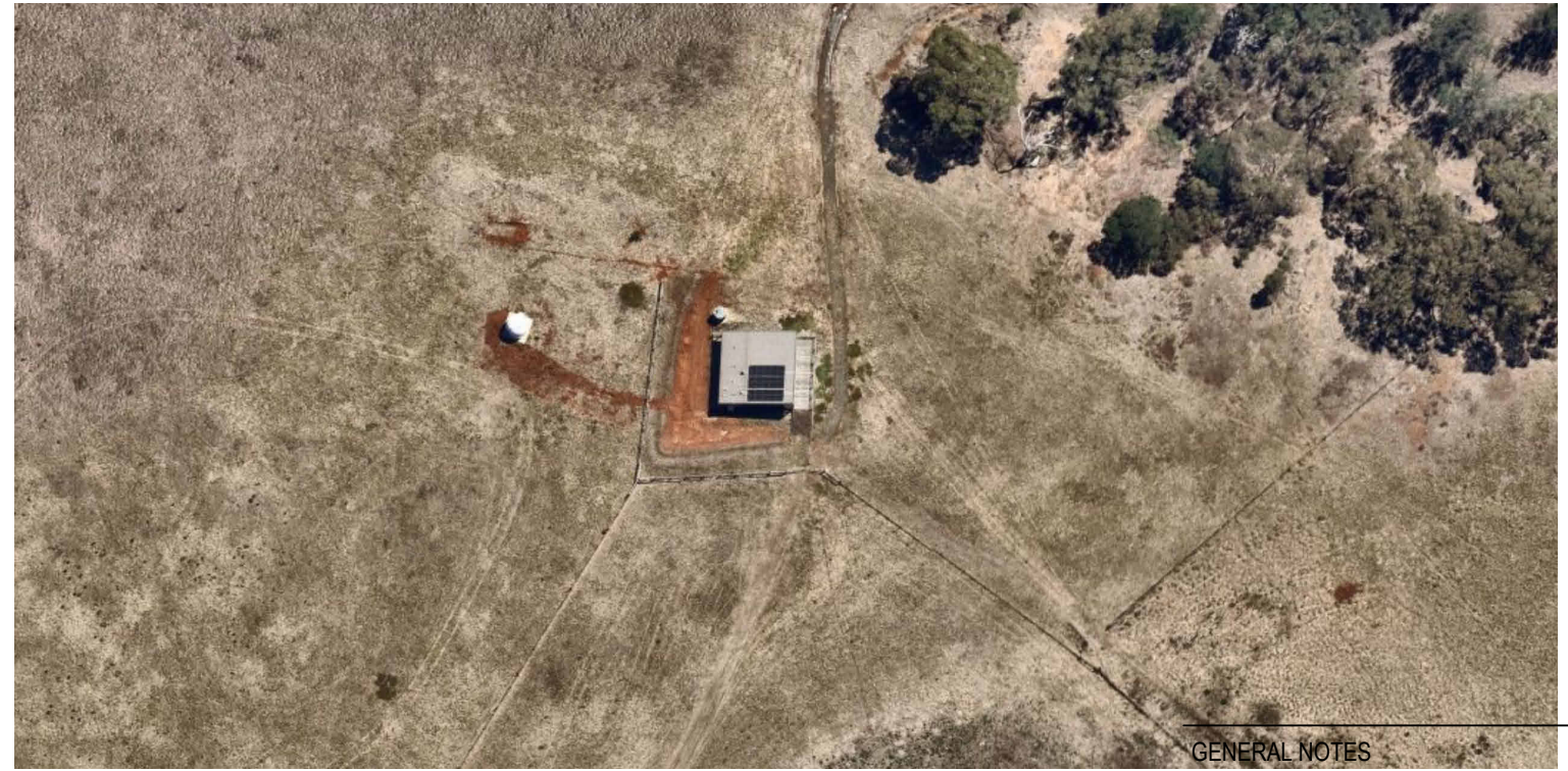
EXISTING SCHOOL BUILDING - OBSERVATION CENTRE
