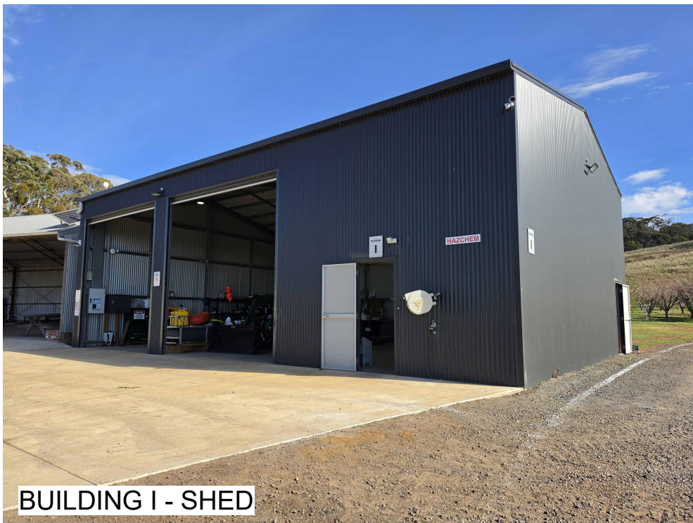
BUILDING I - SHED
