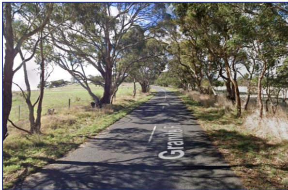
Figure 8: Granite Road – view east
