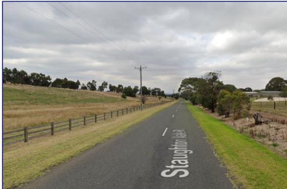
Figure 6: Staughton Vale Road – view northeast
