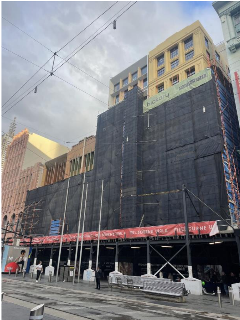
Figure 9 Existing site conditions (October 2024) - Bourke Street frontage
