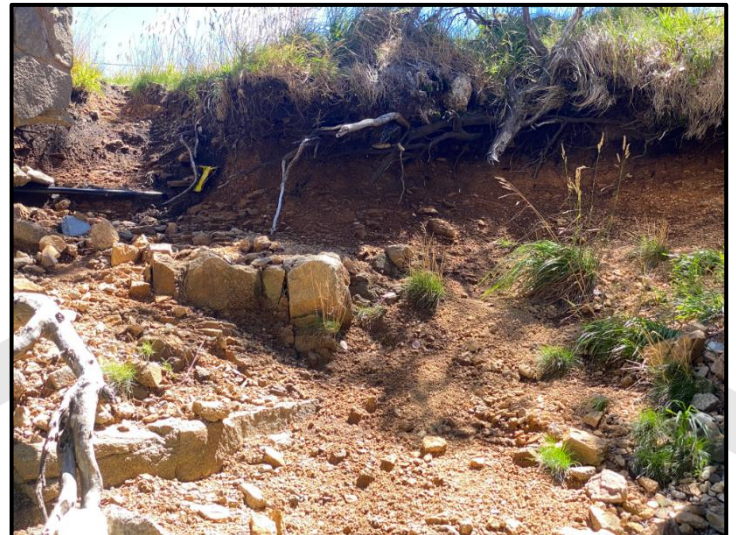
Photo 5 view of typical insitu soil/rock profile exposed in a site cut above Whitehorse Village Road.
