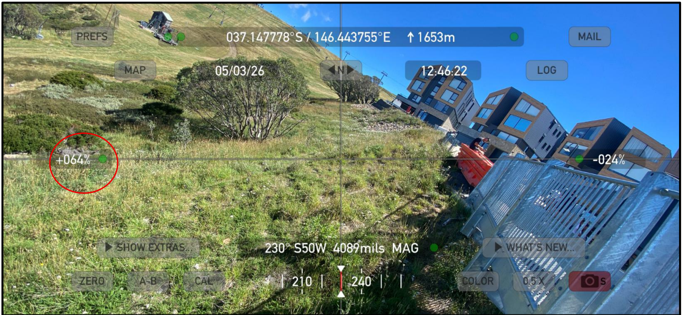
Photo 1 view of typical degree of slope on road fill embankment (taken on angle to match the slope).
