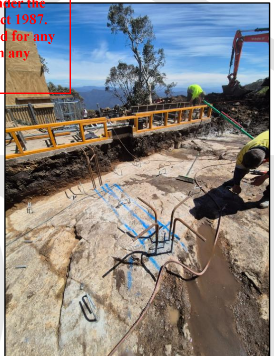
Photo 3 (previously taken by contractor) of insitu, slightly weathered granodiorite bedrock exposed in the footing excavations for that building.
