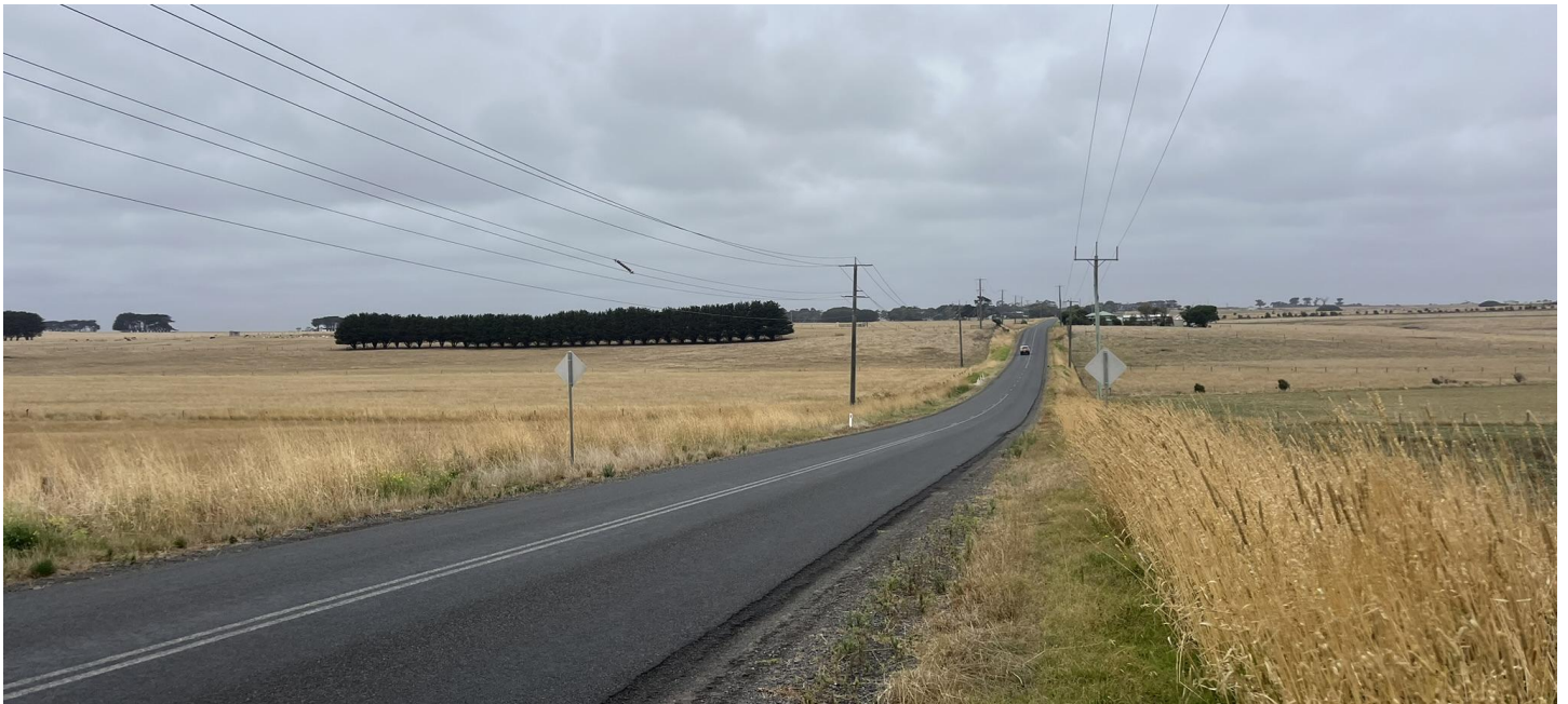
Figure 5: View south along Tower Hill Road. Photo taken on 2 March 2026.
