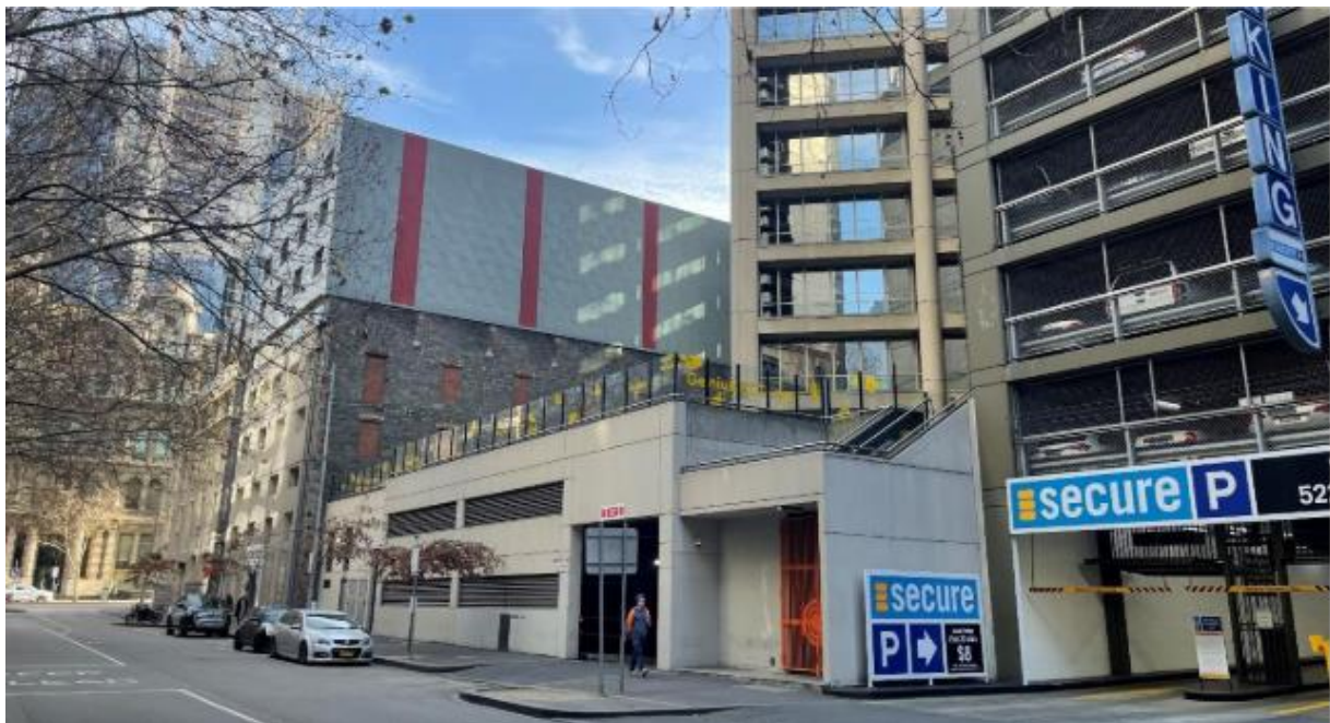
Figure 13 – Existing buildings adjoining the site to the west at 595 Collins Street
