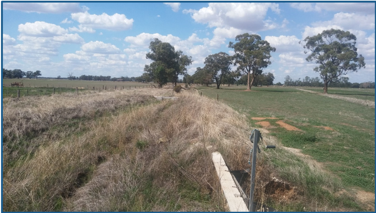
Image 11: The earthen farm irrigation water supply channel in the north-western corner of the site looking east along the northern boundary of the site with an irrigation bay outlet in the foreground, an irrigation channel 'check' at the end of the farm channel and scattered remnant trees in the north of the site in the background.
