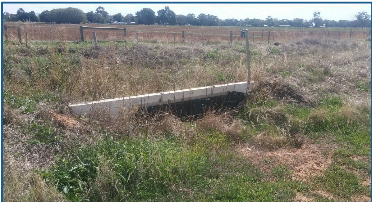
Image 10: One of the fast flow 'Padman' irrigation bay outlets which deliver irrigation water from the farm channel to the irrigation bays
