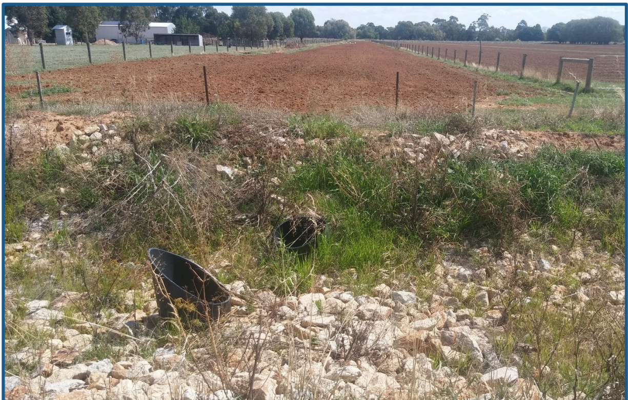
Image 14: Irrigation water is conveyed through a private irrigation water supply pipeline (500m long; 500 mm diameter) from the 6/6 Channel which discharges into a farm irrigation water channel located on a water access easement in the west of the site.
