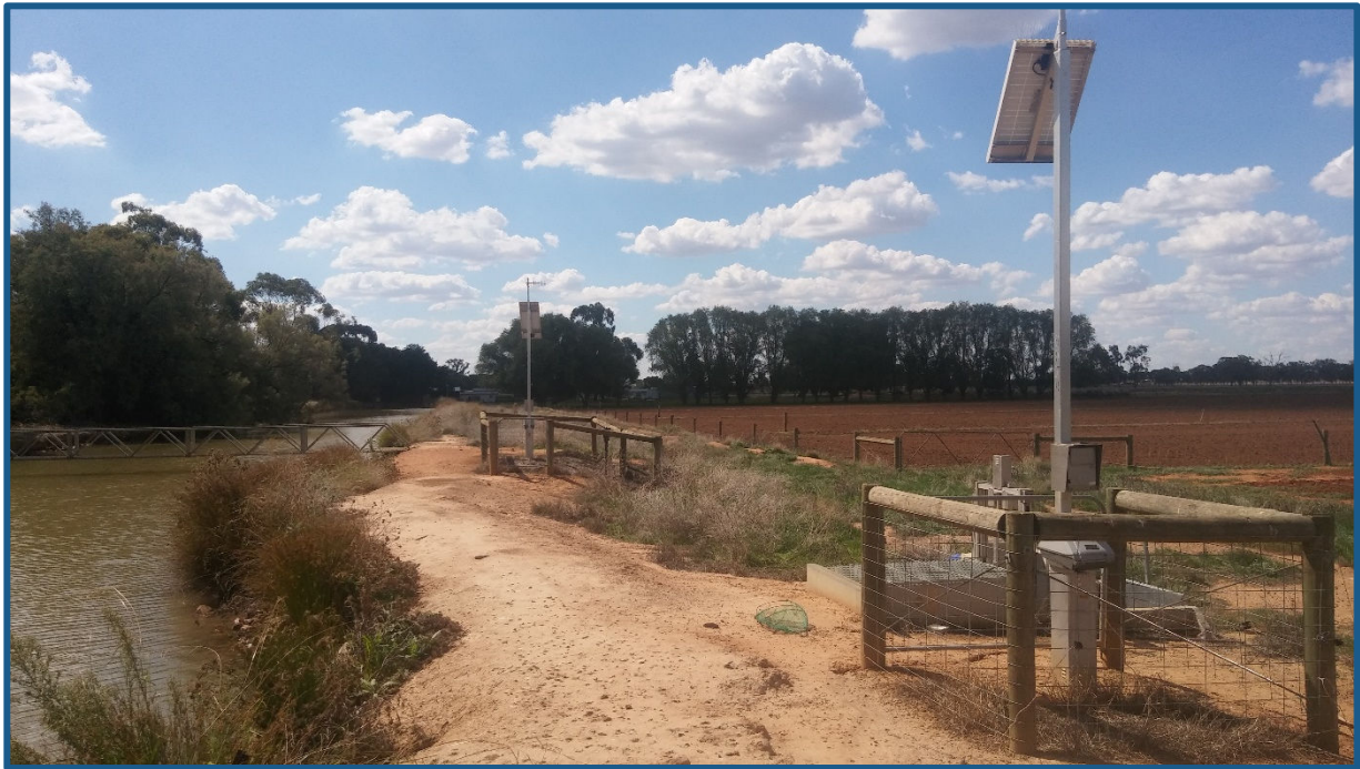
Image 13: Lot 1 is currently serviced by metered outlet MV6071 which is located adjacent to the 6/6 GMW irrigation channel approximately 500 metres west of the site.
