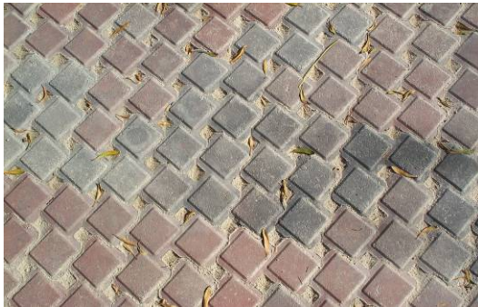
Detail of Rocla Ecotrihex® as laid showing gaps between the pavers filled with propagation sand.
