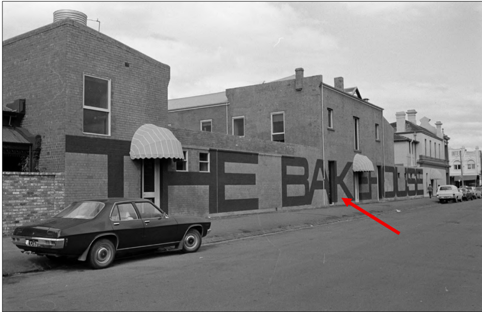
Figure 6 Subject site c.1970 showing the bake house, stable and low connecting building, still of face brick at this time. As seen in figure 8 below, an additional door has now been inserted where indicated by the red arrow and the windows all replaced. Source: Committee for Urban Action, SLV http://handle.slv.vic.gov.au/10381/4154490
