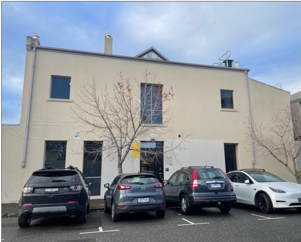
Figure 8 The Erskine Street elevation to the former bake house. With its rendered surfaces, additional door opening and modern glazing, it is a much altered structure.
