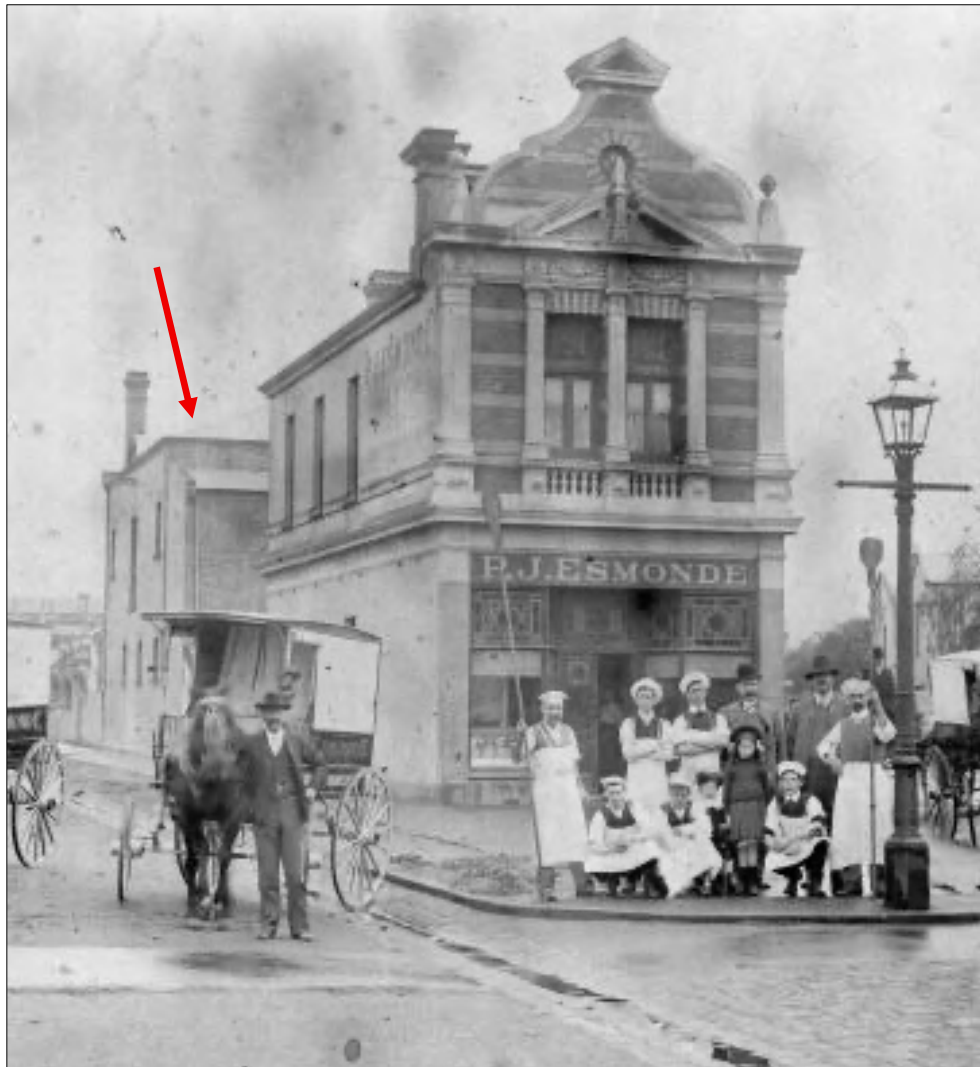
Figure 2 The P J Esmonde bakery viewed from Armstrong Street, 1908. The bake house on Erskine Street is visible to the left (marked by the red arrow). Source: Port Phillip City Collection
