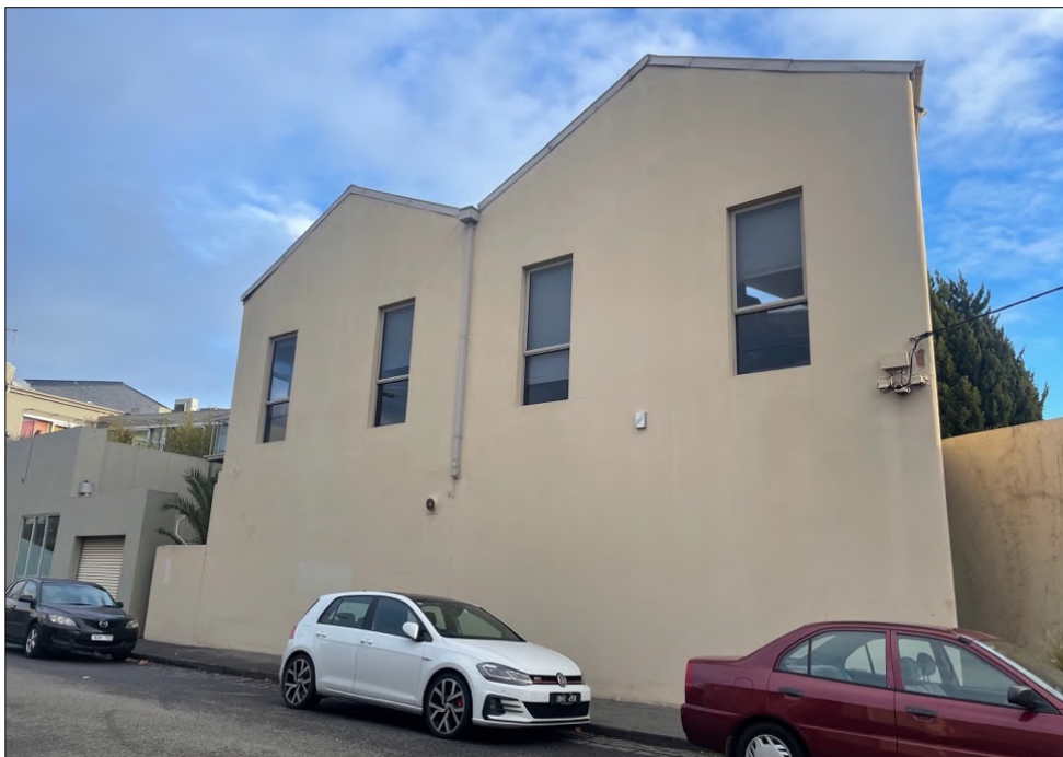
Figure 16 Canterbury Place elevation of the double storey, double gabled bake house additions, understood to date to the late interwar period. Like the other envelopes, the face brick has been rendered.
