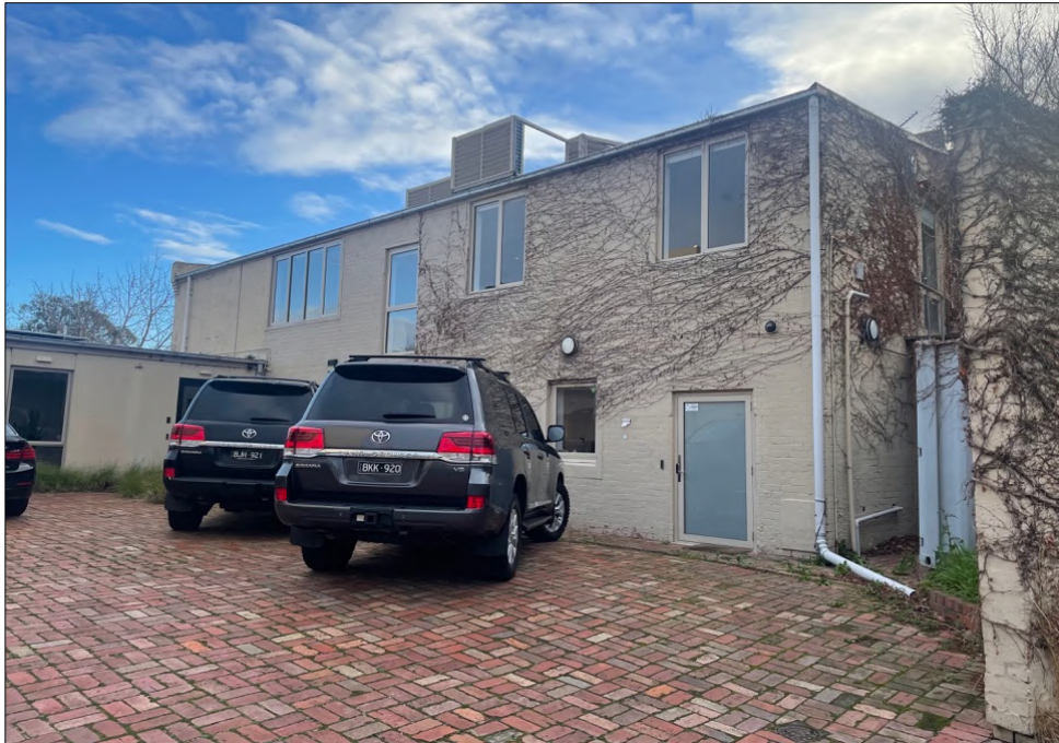
Figure 19 Eastern elevation of the former stable. The openings to this building have been altered and the brickwork to this elevation painted, and it retains little of its original character.
