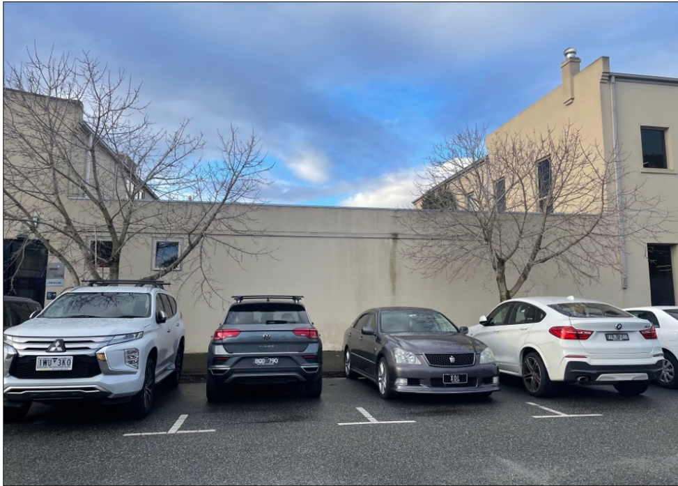
Figure 9 The central building envelope within the site, connecting the former bake house to the former stable. This is understood to have been constructed c.1970.
